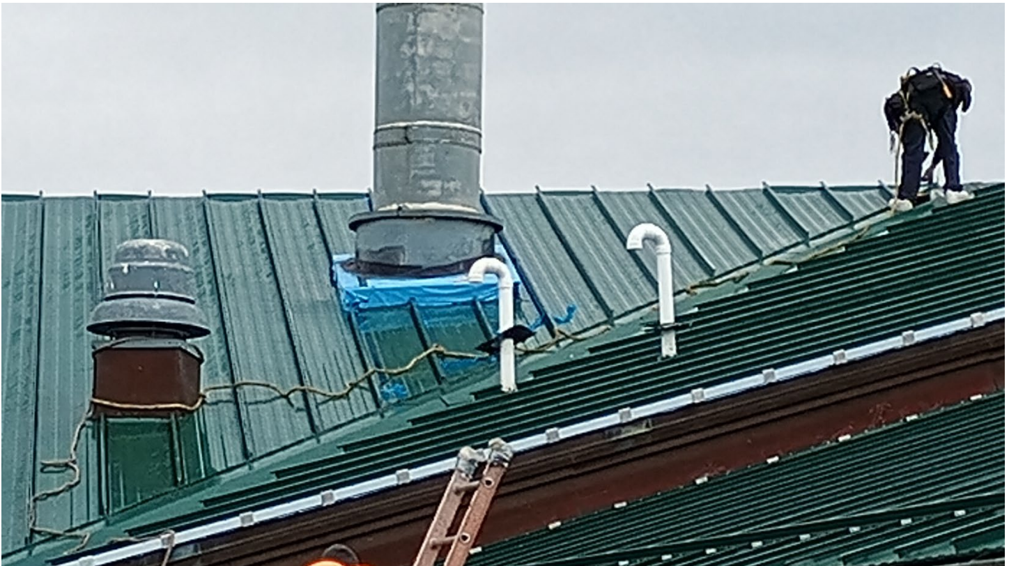
Roof E – Box out of roof exhaust
