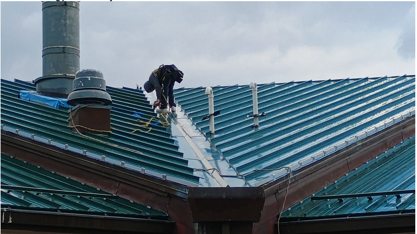
Roof E – Securing panels to valley
