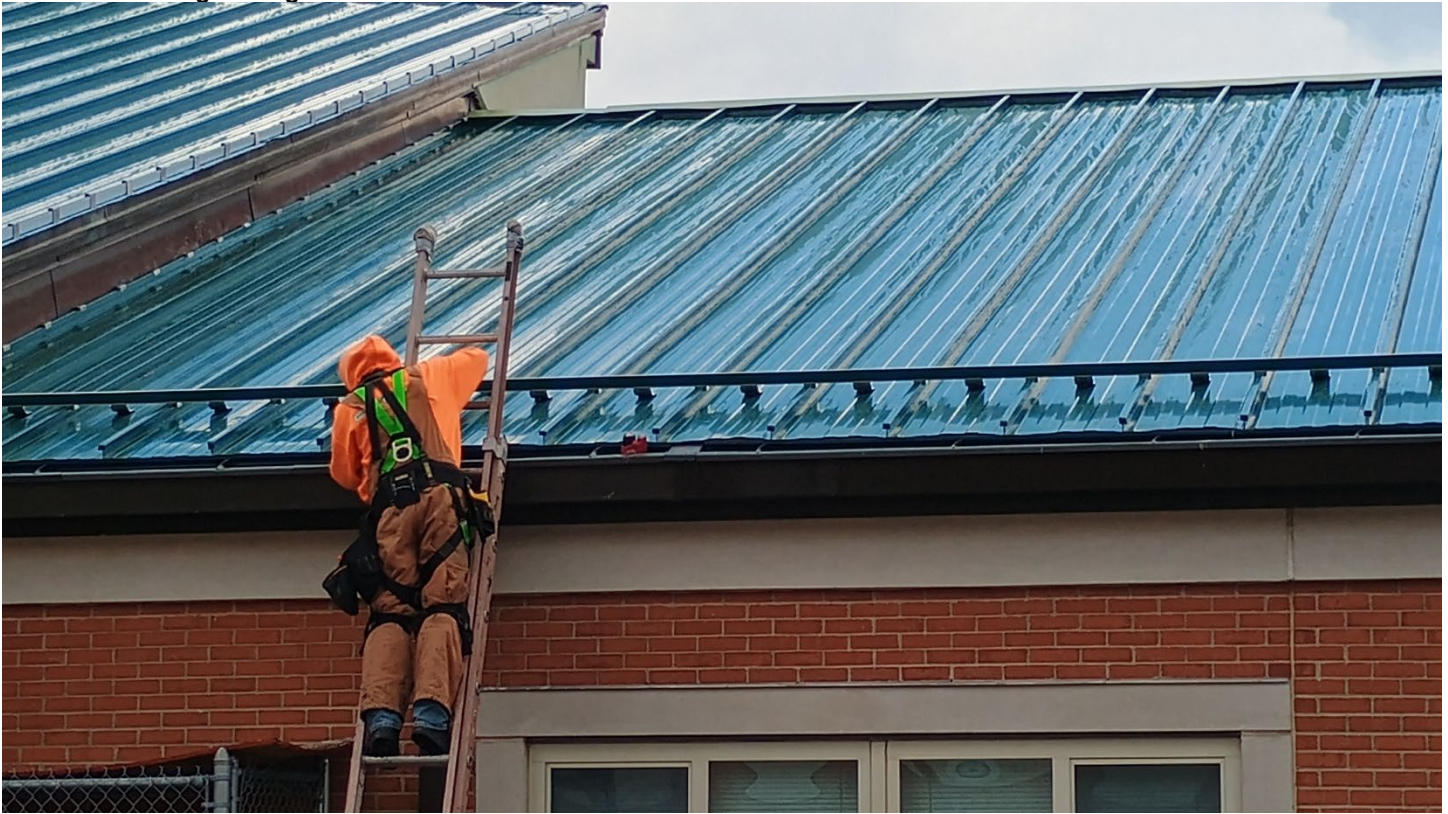
Roof F – Installing snow guards
