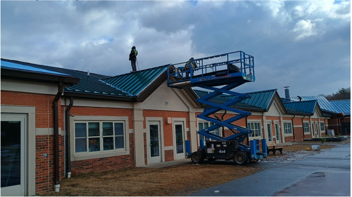
Roof D – Ridge work in progress
