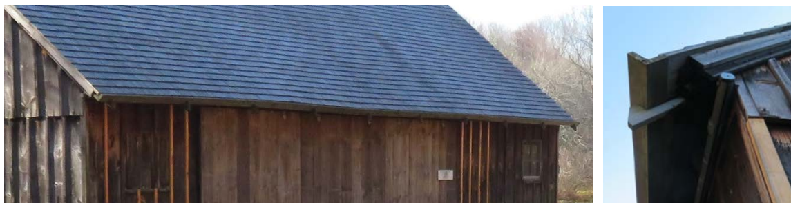
North gutter overall and profile of V-shape and bracket.
