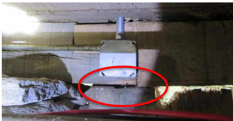
Top: East wall post from south and west respectively; Bottom: gap between top of post and beam/sill.
