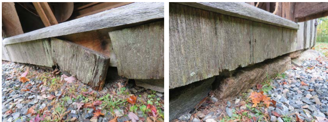
Siding and foundation below grist mill exterior doors. Siding nails have failed, but sill behind appears to be in good condition.
