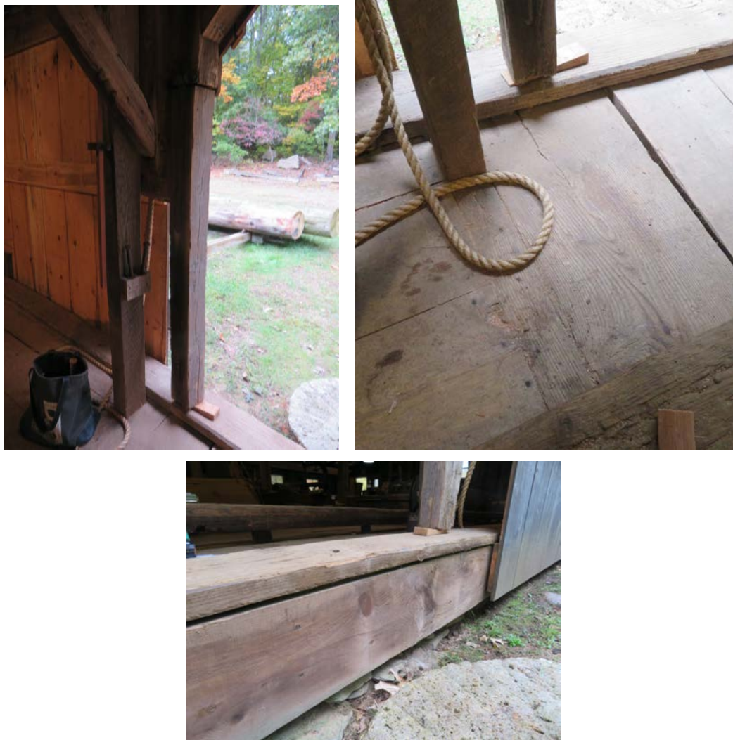
Loft-west, north post. Top: “new” offset post overall and zoomed in view at base supported by decking as well as deflection of deck board relative to adjacent one; Bottom: exterior view showing gap between door sill and skirt board suggesting lifting of door sill by decking.
