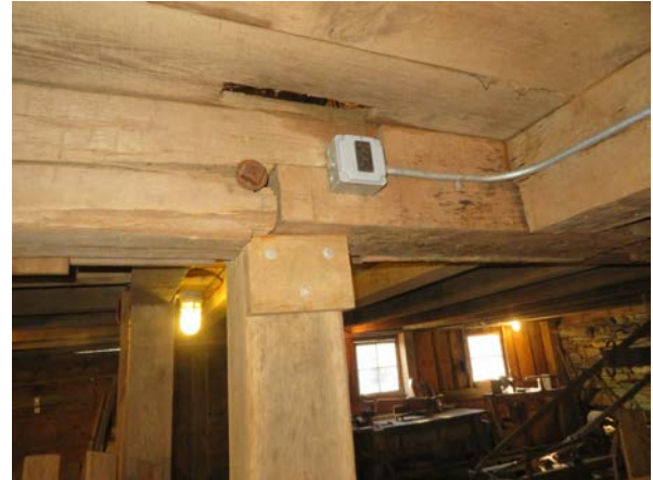
Left: from the southwest showing ledge, board siding and original building sill/beam with deep vertical check, as well as ledger on post to support inner edge of beam; Right: from north showing bolted lap splice over post, split, and ledger on post.
