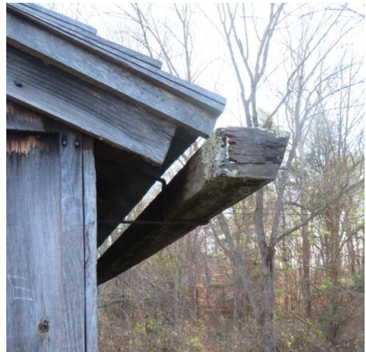
South gutter showing dip (likely missing bracket) toward east end.
