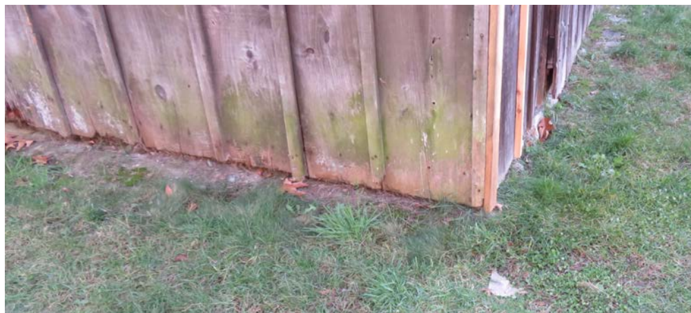
Biological growth, weathering, deterioration and replacement battens (shown at northwest corner).
