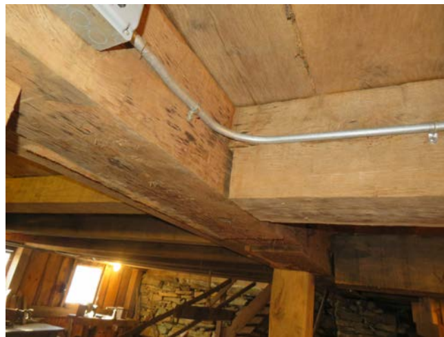
Shear crack in original mill joist framing into the sill / beam (behind the conduit).
