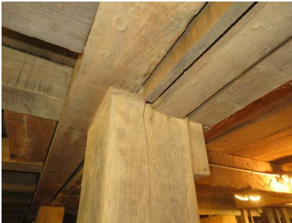
Left: from the southwest showing ledge, board siding and original building sill/beam with deep vertical check, as well as ledger on post to support inner edge of beam; Right: from north showing bolted lap splice over post, split, and ledger on post.
