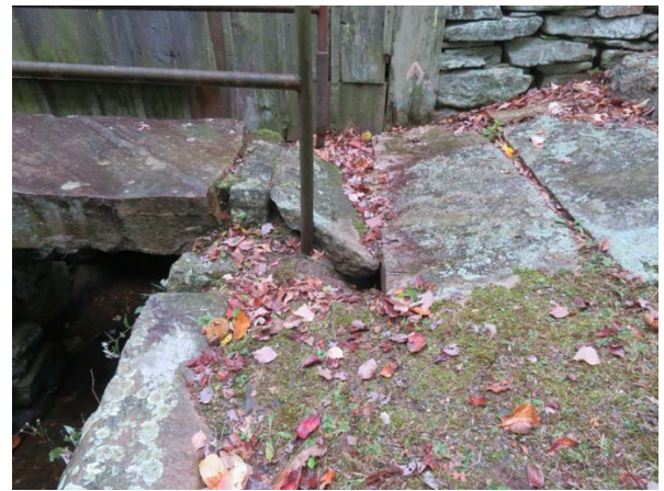
Top: Overall view of damage; Bottom Left: Bulge in foundation wall; Bottom Right: Shifting and movement of bottom 3 steps due to erosion of soil below.
