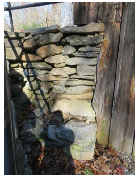
Displacement of steps and dry laid retaining wall at lower level below eroded areas above
