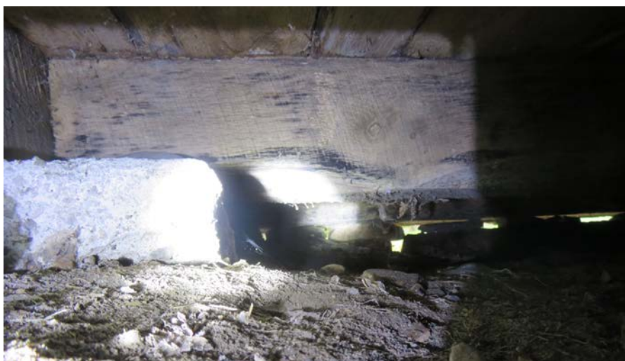
East end of joist in grist mill floor (crawl space) showing black staining and close proximity to grade, but not visible deterioration.
