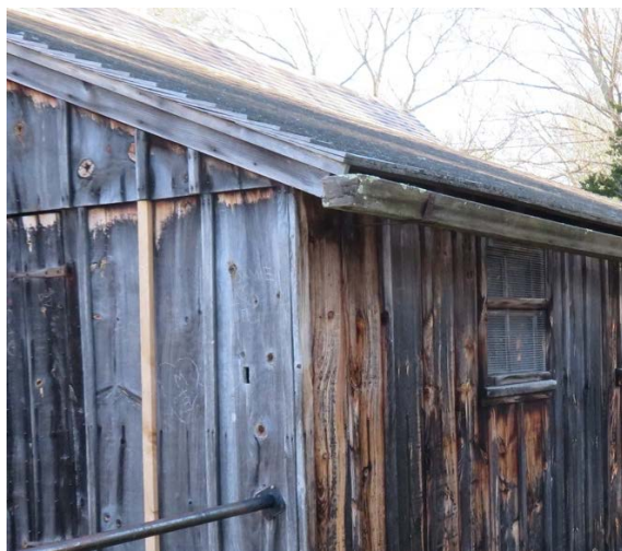
South gutter showing dip (likely missing bracket) toward east end.
