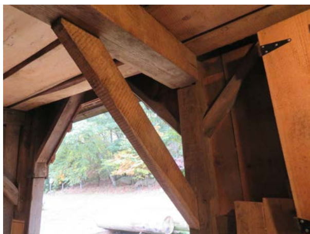
Loft-Central support line. Top: Middle post and beam connections at top; Middle: Middle post connection at bottom; Bottom: Beam connections into end post using historic joinery.
