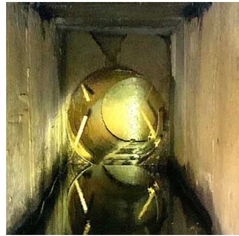
Left: investigation of the gate showing structure behind gate assembly; Right: concrete culvert between grate and penstock (penstock beyond). Both images courtesy of Ledyard Up-Down Sawmill Facebook page.
