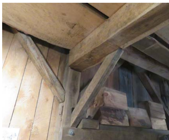
Loft-Central support line. Top: Middle post and beam connections at top; Middle: Middle post connection at bottom; Bottom: Beam connections into end post using historic joinery.
