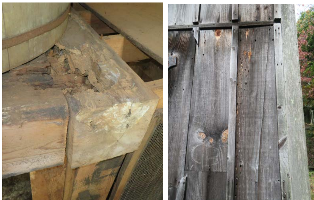
Left: Termite damage at the grist mill frame; Right: tell-tale termite trails / holes at siding at the east end of the south elevation.
