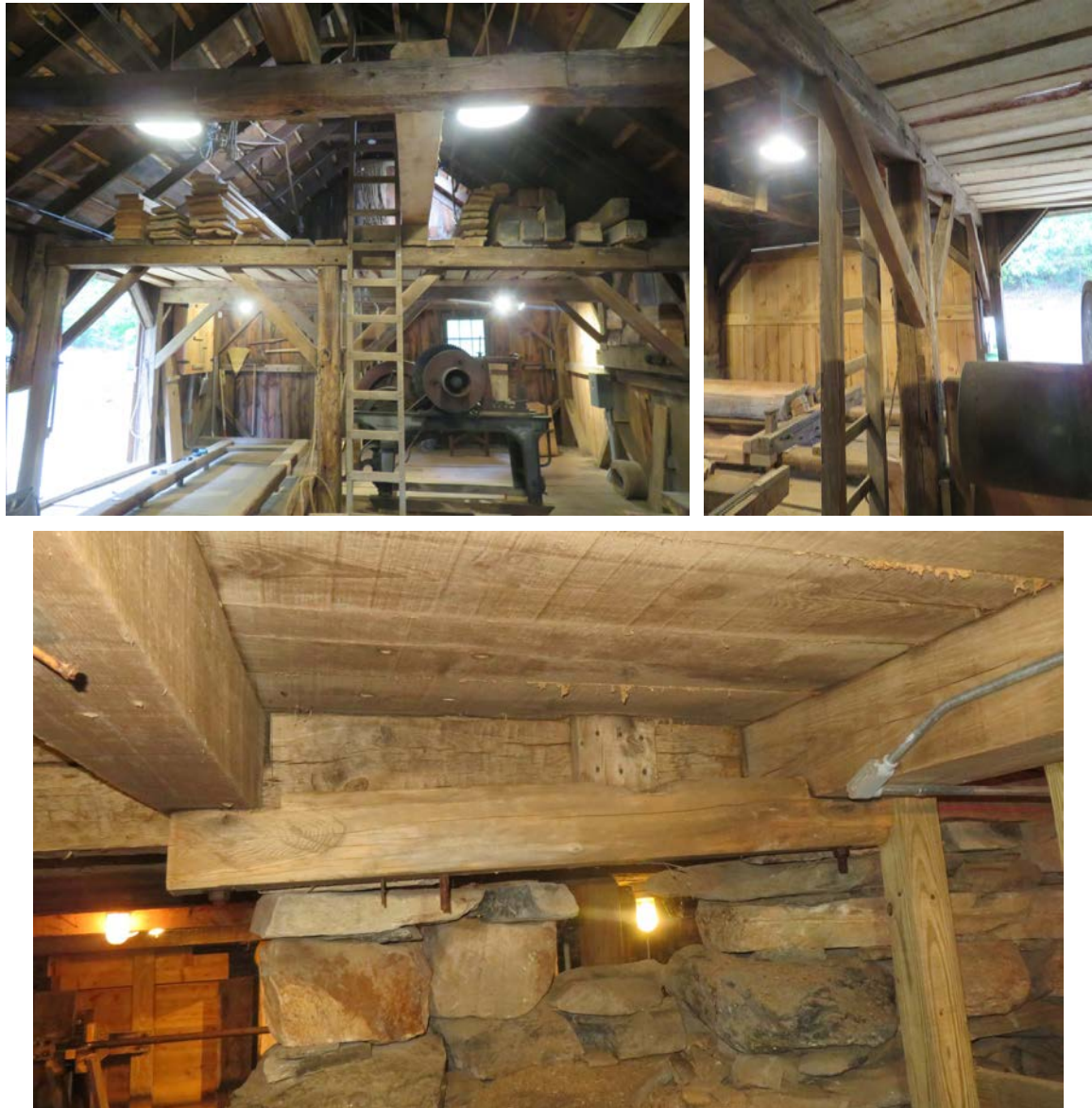
Overall Loft and Loft-West support line. Left: Loft-West north bay showing replacement post; Right: Loft-West middle post with hung beam support below.
