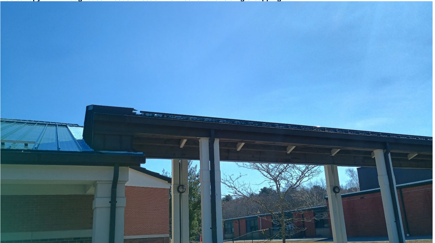
Bus canopy – Mini “doghouse” needs direction from Garland for siding & capping
