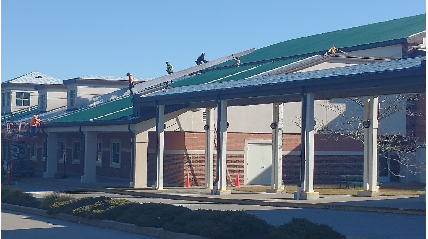
Roof A – installing metal panels on the western elevation
