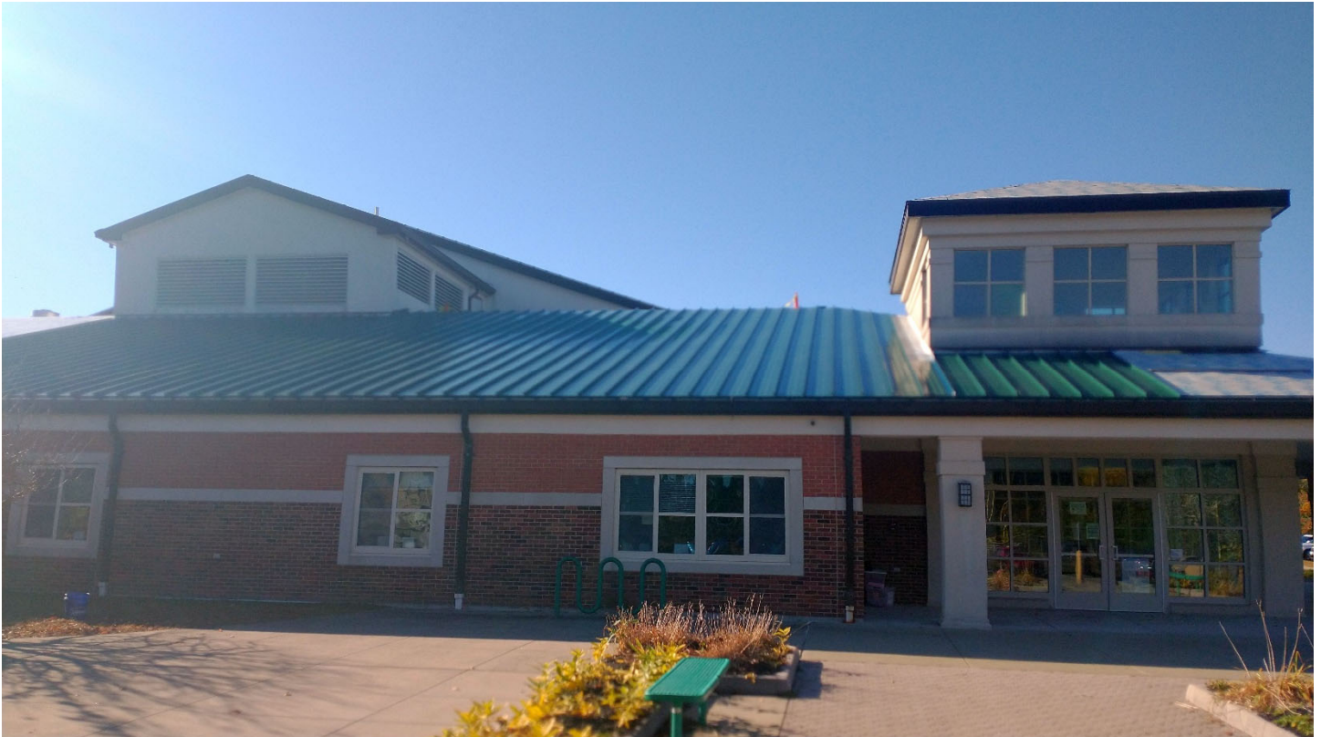
Roof A – North elevation
