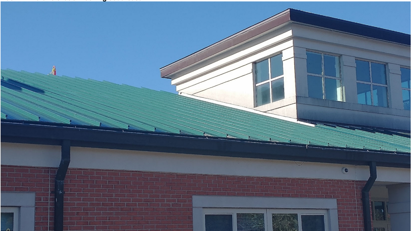
Roof A – North elevation looking southeast
