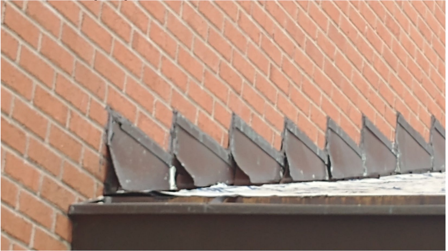
Roof A – Reviewed flashing, looks good.
