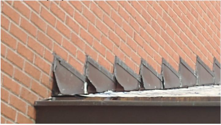
Roof A – Peel & stick has been laid, waiting on roof panels
