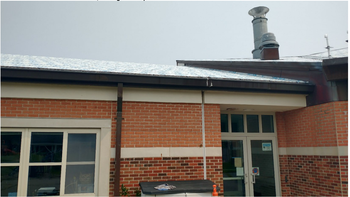
Roof D – Peel & stick has been laid, waiting on roof panels
