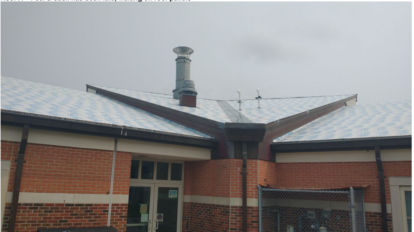
Roof A – Peel & stick has been laid, waiting on roof panels
