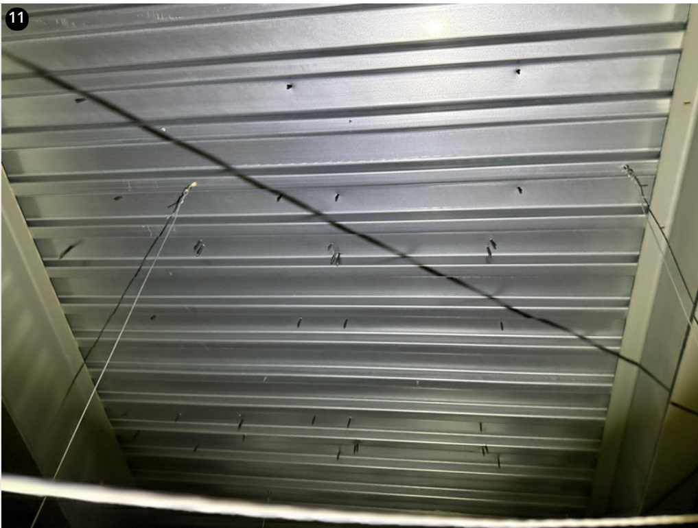
Proper deck fastening pattern with 8" fasteners
