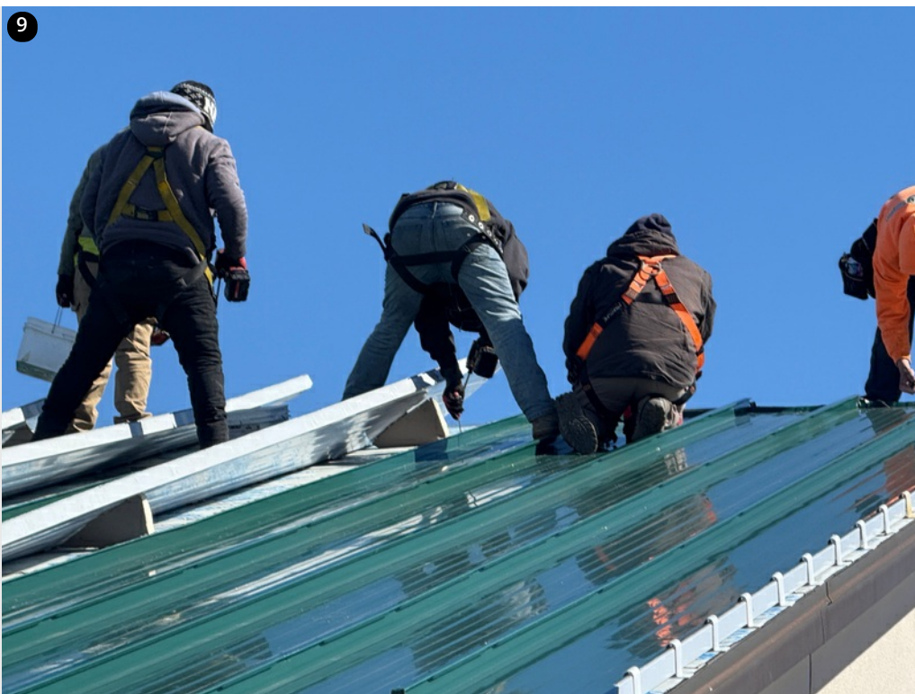
Replacing fasteners with 8" HD's
