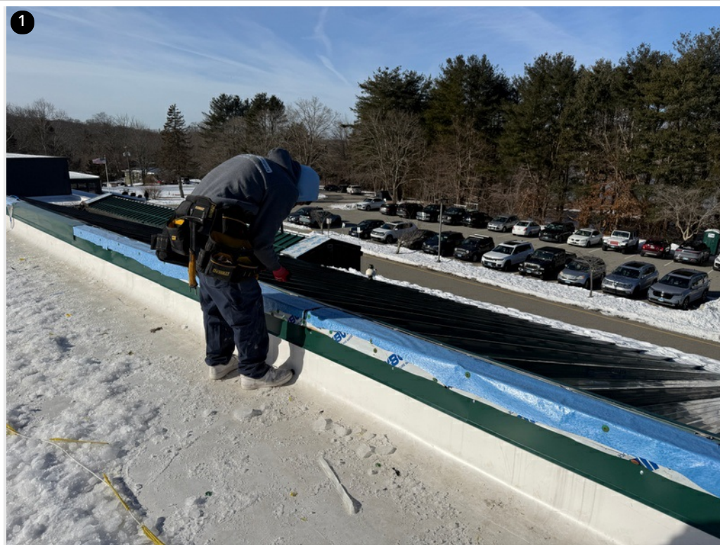
Working on the low slope to slope head detail
