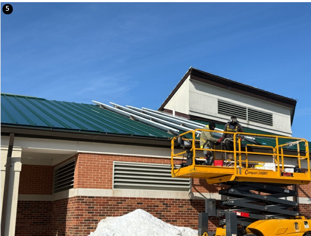
Crew starting fastener replacement on the back of the kindergartener wing
