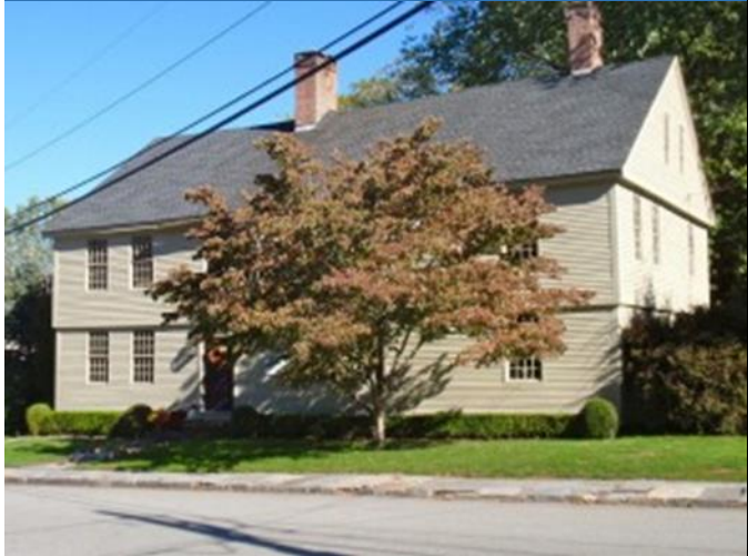
Simon Huntington House, c. 1690 (enlarged 1760 and 1780) 2 Elm Ave
