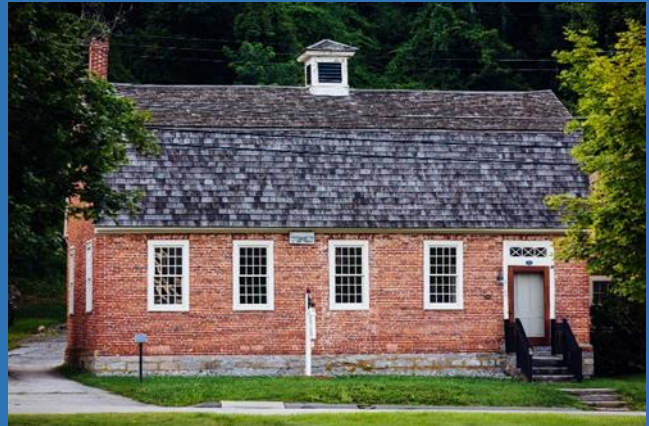
Lathrop Schoolhouse, c. 1783 69 East Town Street
