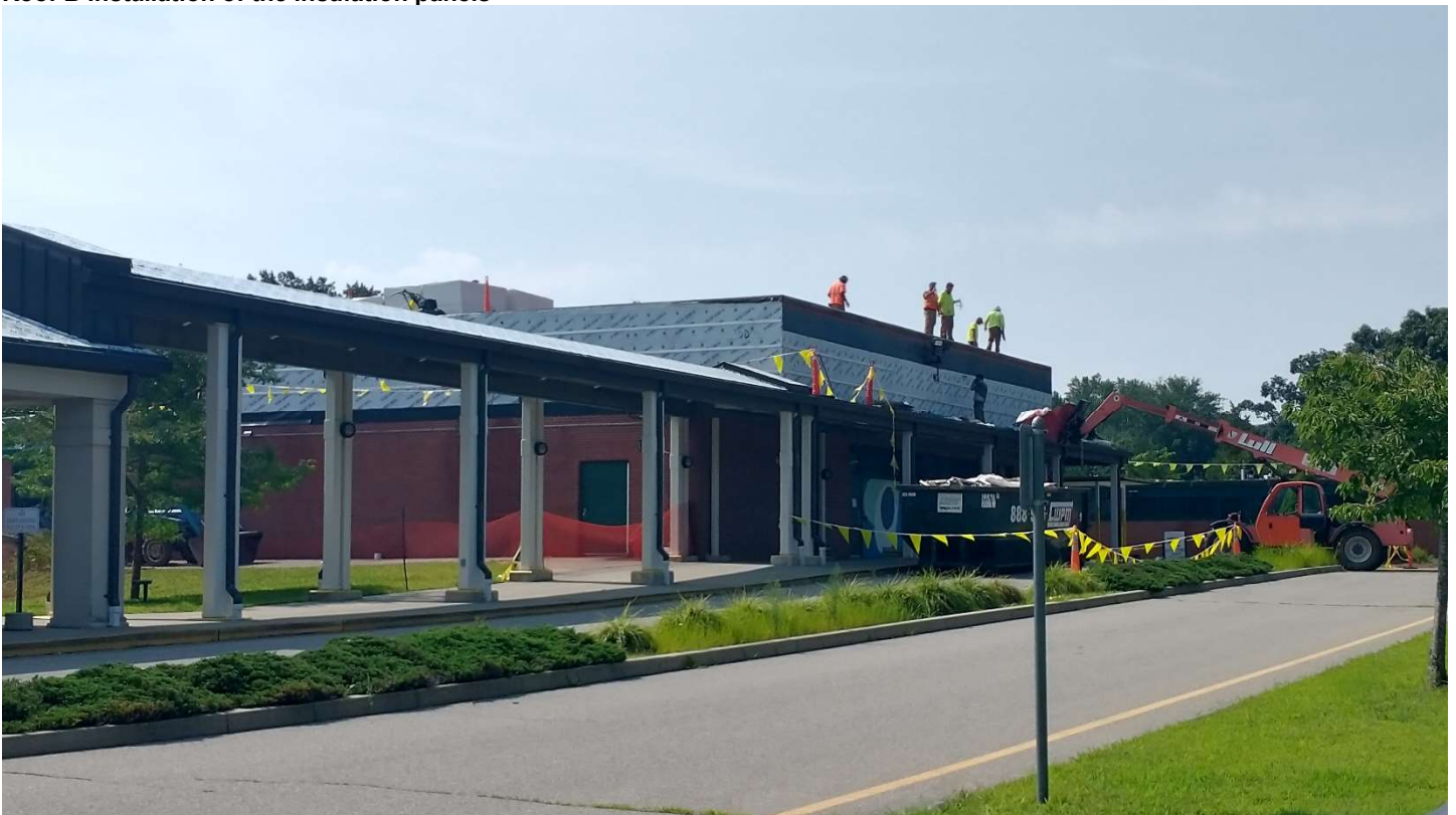
Roof B installation of the insulation panels
