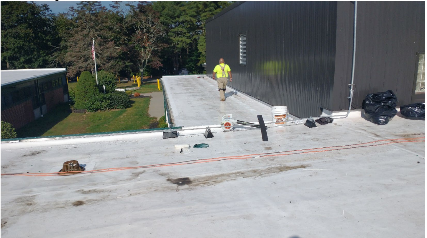
Roof D – Looking east
