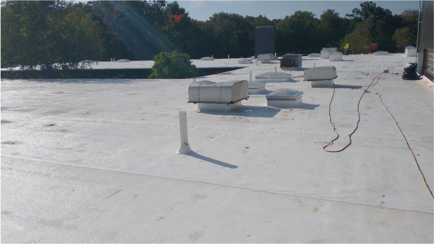
Roof A – Looking South
