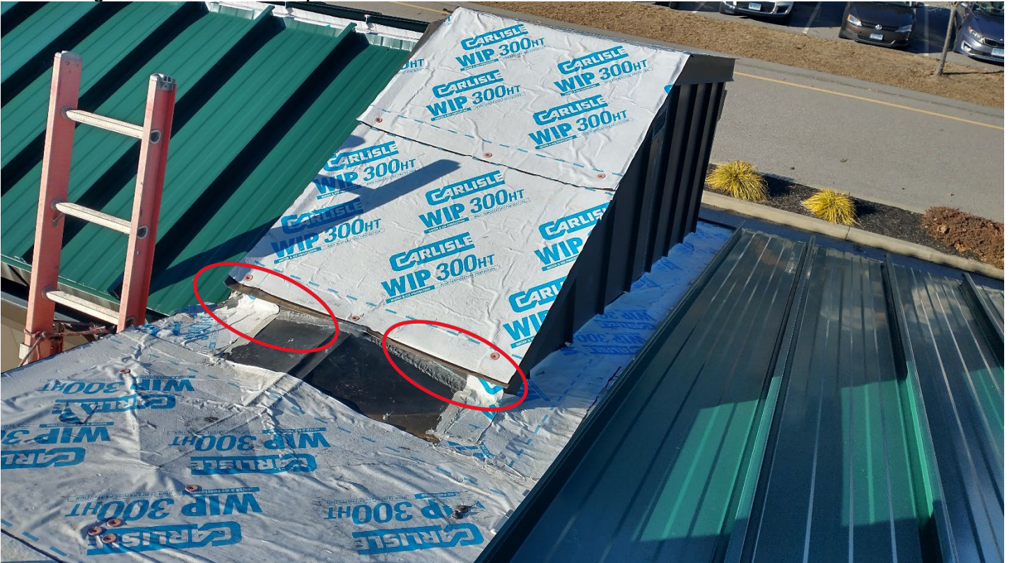
Roof A – In garland's hands to come up with a solution for the cricket due to vertical side walls on both sides of the cricket
