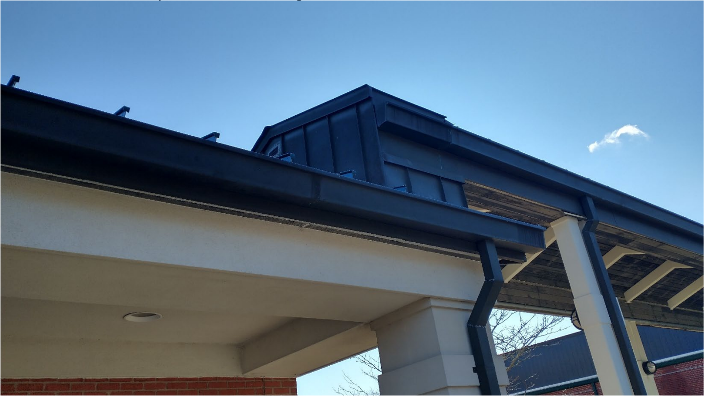
Roof A – Discussed vertical panel installation on the gable end
