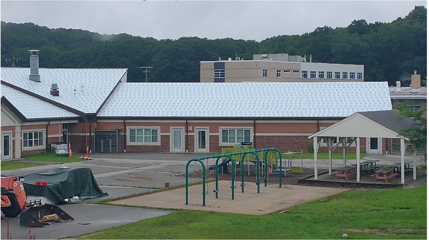
Roof F – Peel & stick has been laid, waiting on roof panels
