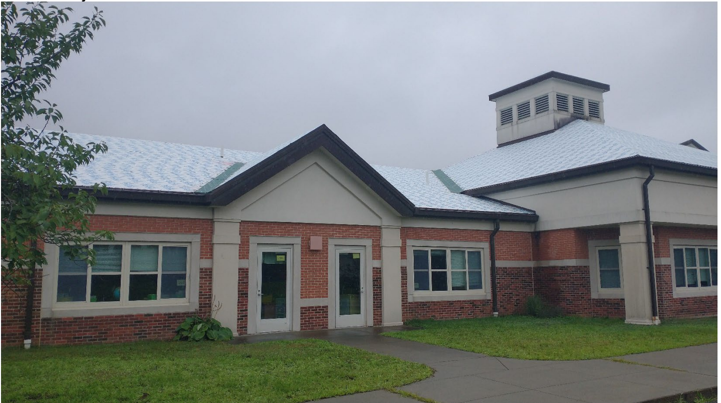
Roof D – Valley work
