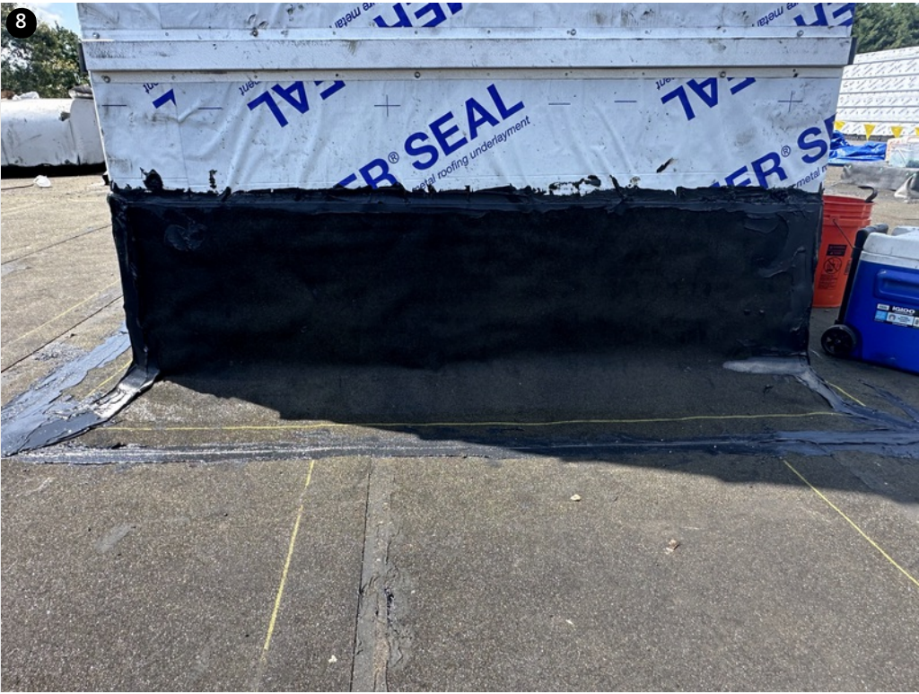
8 Base flashings around chimney- Proper height- No open corners or seams
