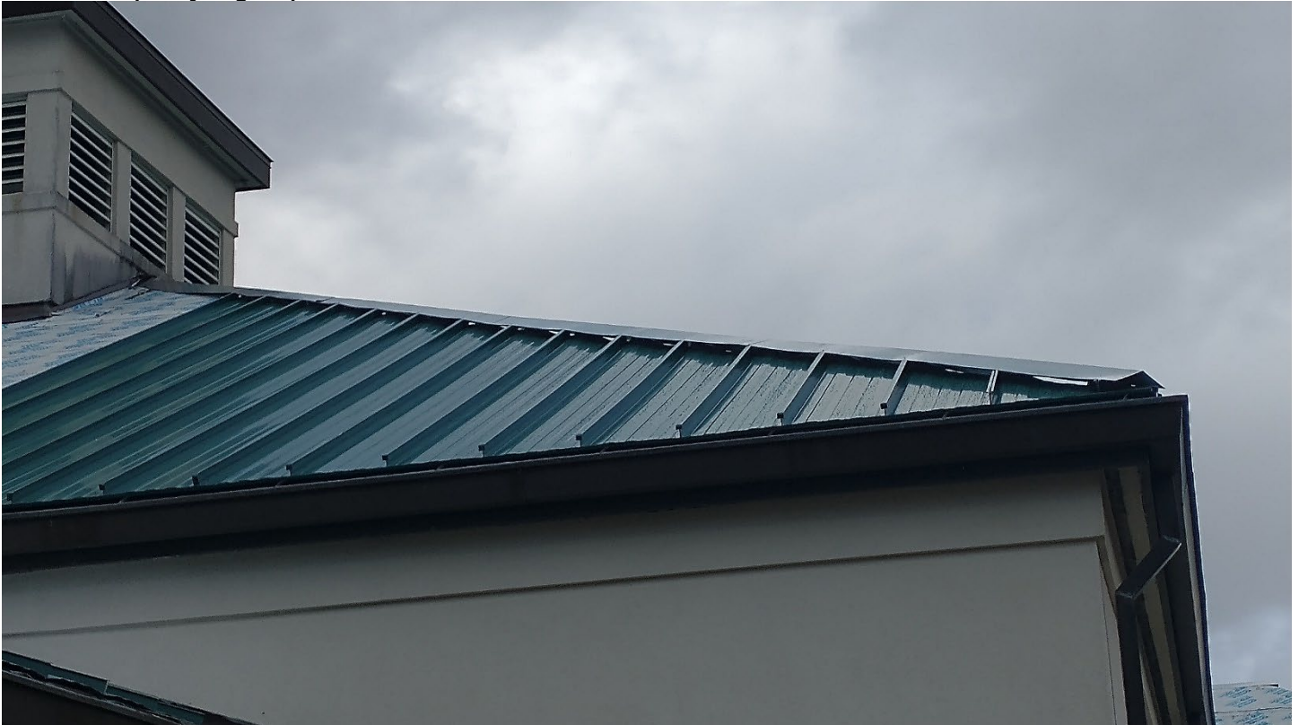
Roof A – temporary ridge caps
