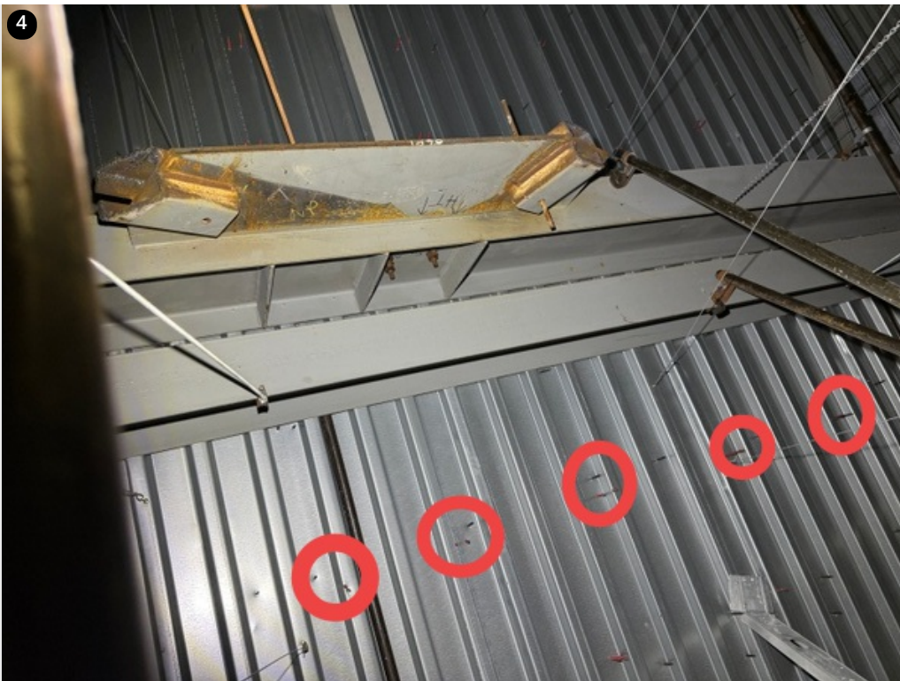
Fasteners observed penetrating deck- 1/6/25
