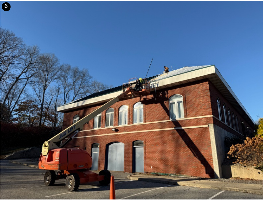
Crew installing panels on back section- 11/19/24
