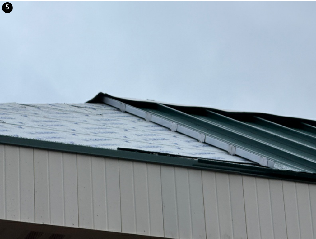
Clips fastened and spaced at 1' 8" throughout- 11/19/24
