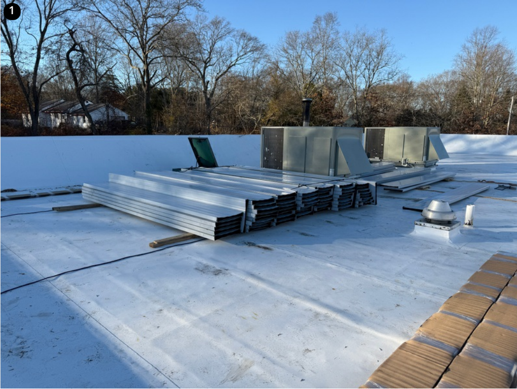
Panels loaded onto roof and prepped for installation- 11/18/24
