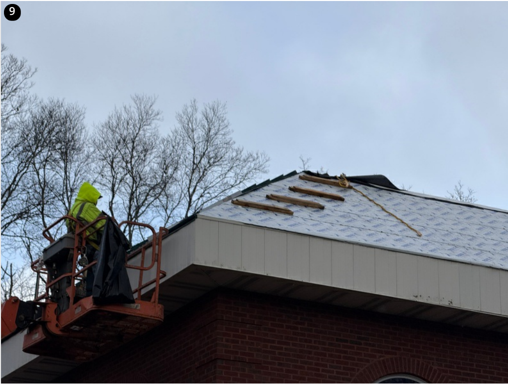
Crew installing panels on back section- 11/22/24
