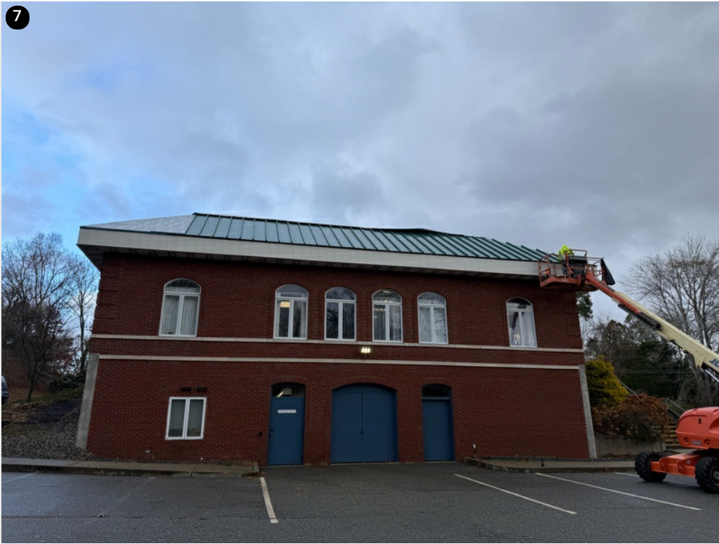
Crew installing panels on back section- 11/22/24
