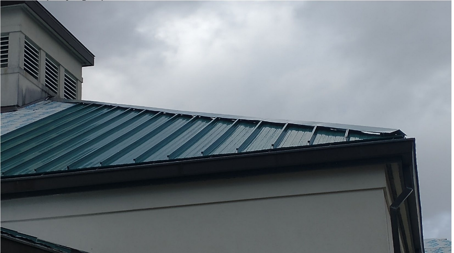
Roof A – temporary ridge caps
