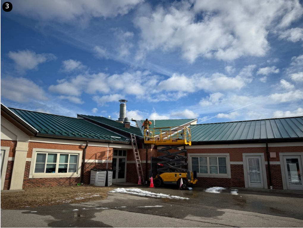
Crew installing panels on the boiler room section- 2/4/25
