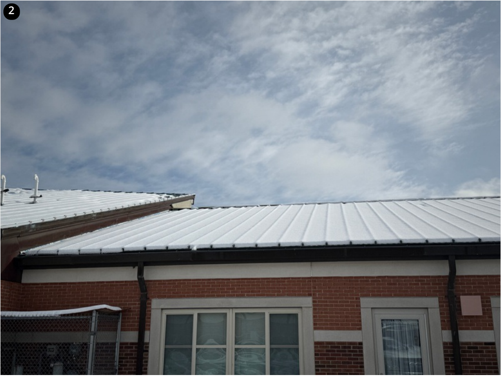
2 Panels installed over the weekend on Kindergarten wing- 2/3/25
