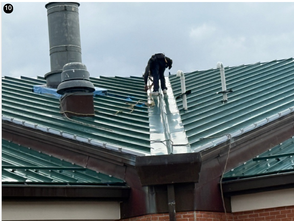
Crew riveting panel ends on boiler room section- 2/7/25
