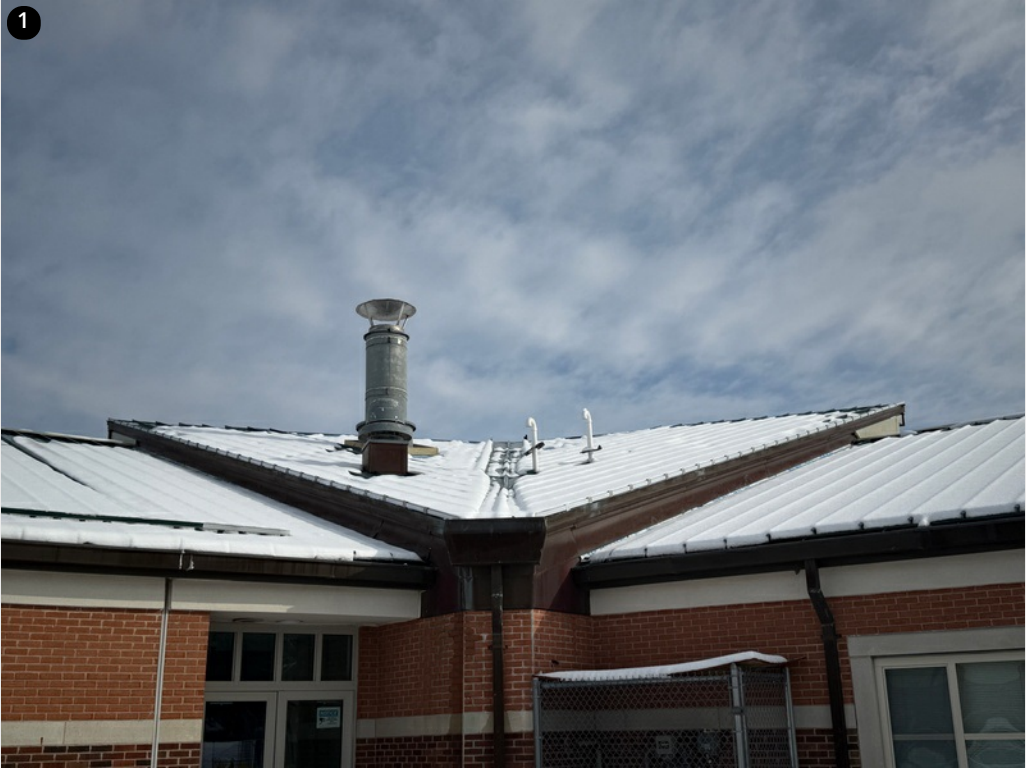
1 Overview- Boiler room section progress- 2/3/25
