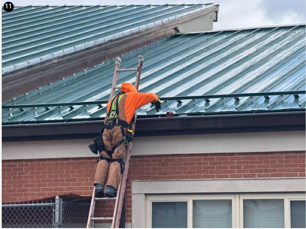
Crew riveting panel ends over Kindergarten wing- 2/7/25
