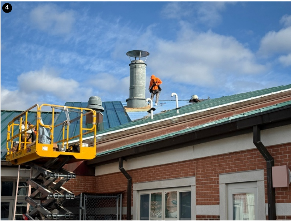
Crew building curb around stack penetration- 2/4/25
