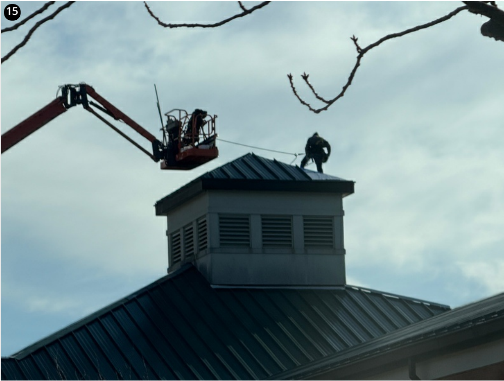
Crew installing panels on small copula- 1/16/25
