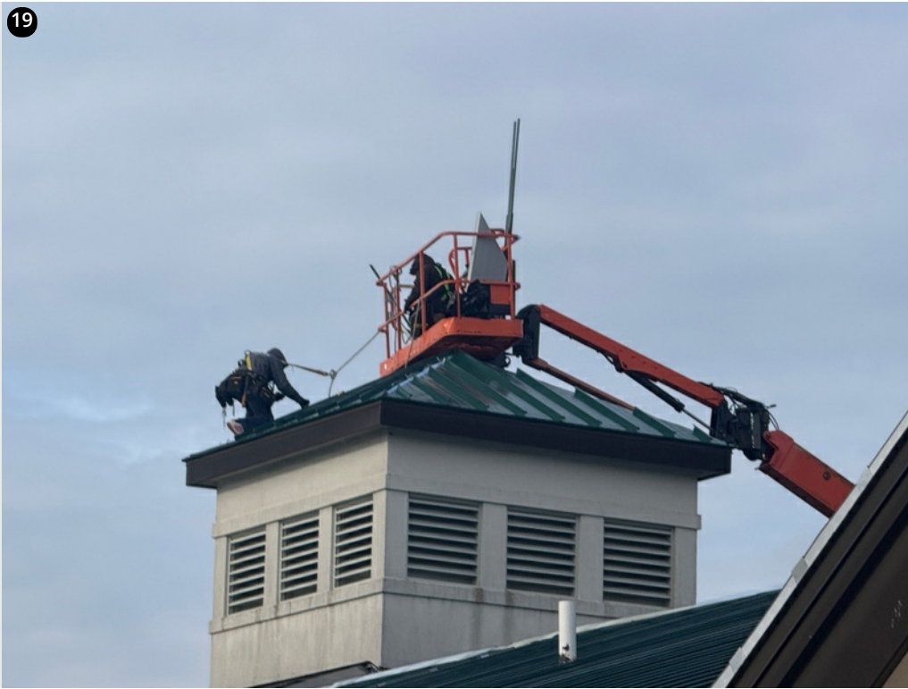
Crew installing panels on small copula- 1/17/25
