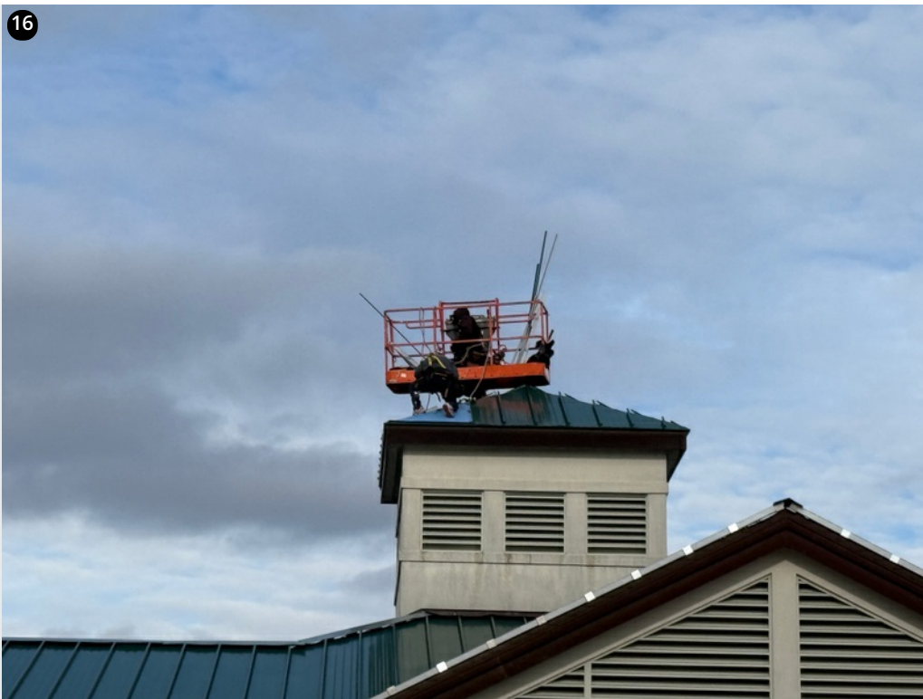
Crew installing panels on small copula- 1/16/25
