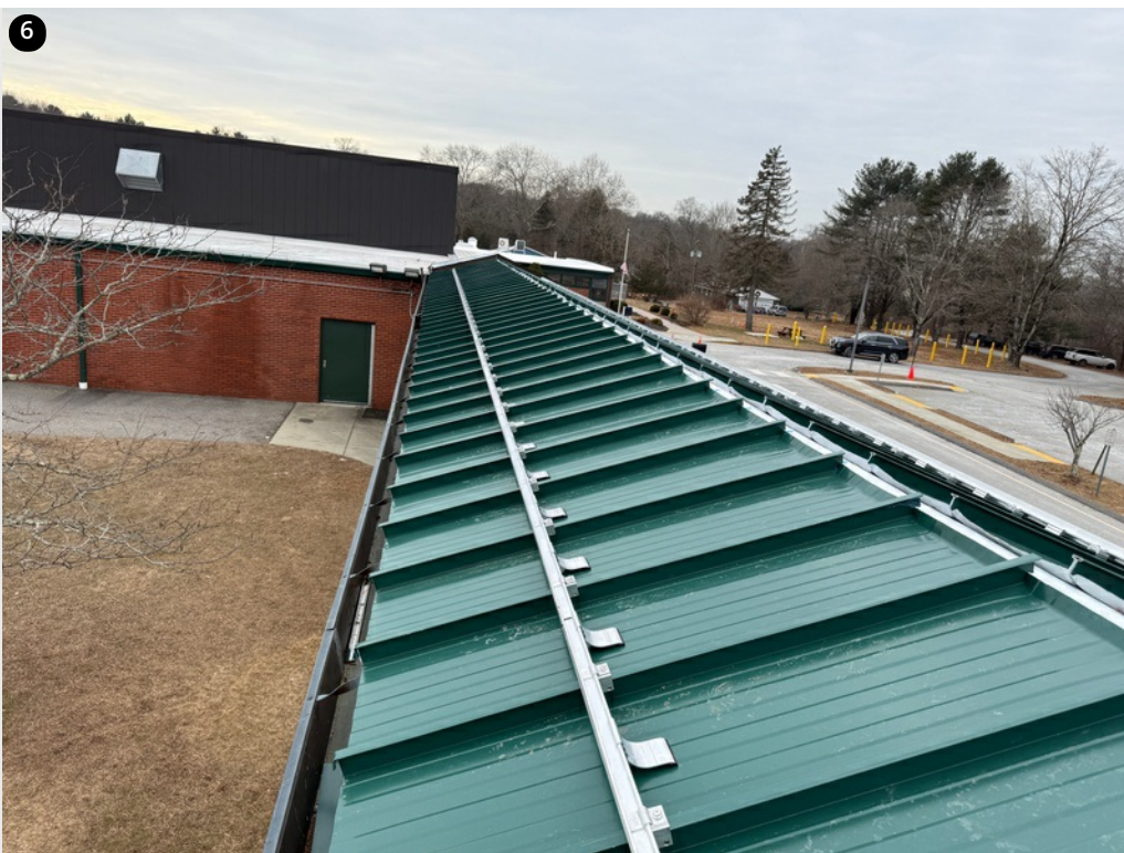
Snow guards installed on walkway roof- 1/13/25
