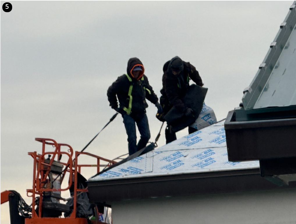
Crew removing loose and expired ice and water layer on small copula- 1/13/25
