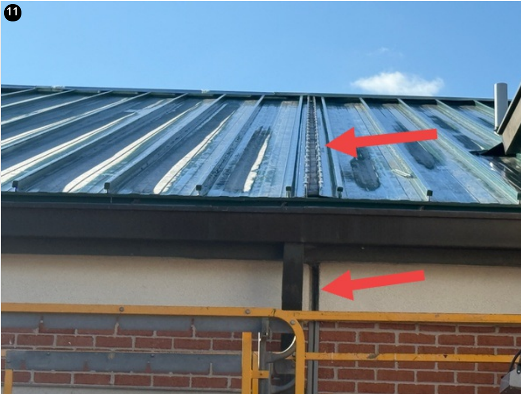
Gable clips installed on both sides of expansion joint- 1/14/25
