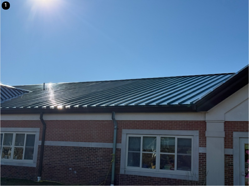
Panels installed Saturday 11/23/24
