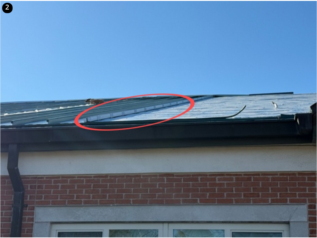
Panels installed Saturday 11/23/24
