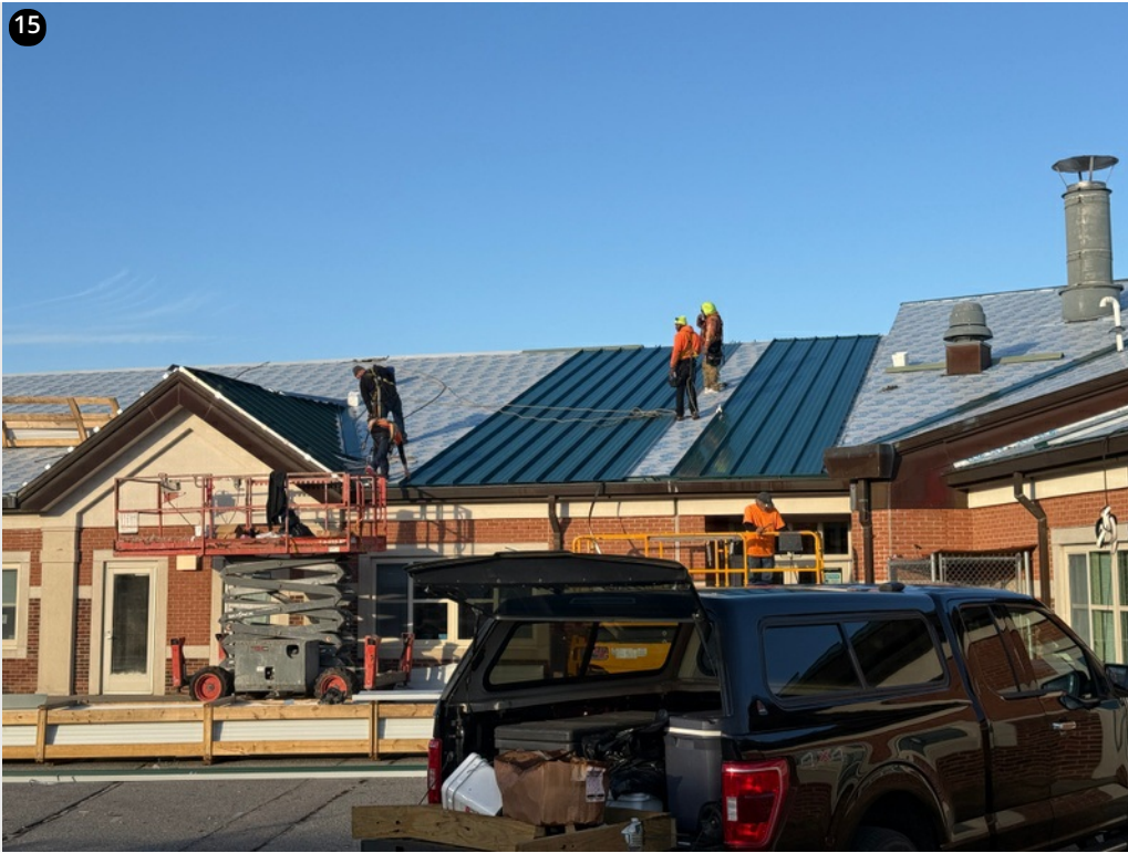
Half of dormer completed- Panels installed on field section- 11/27/24
