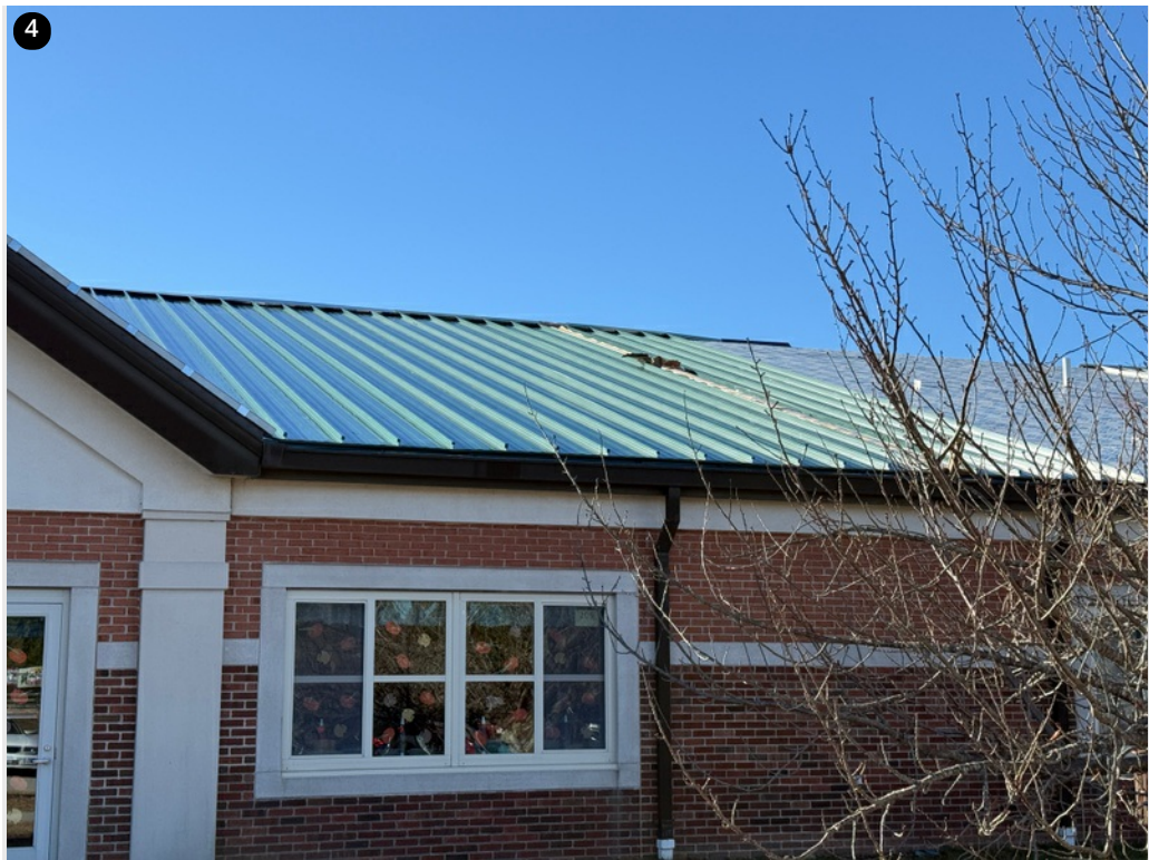
Panels installed Saturday 11/23/24
