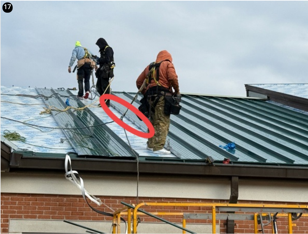
Crew installing panels on field section- 11/29/24
