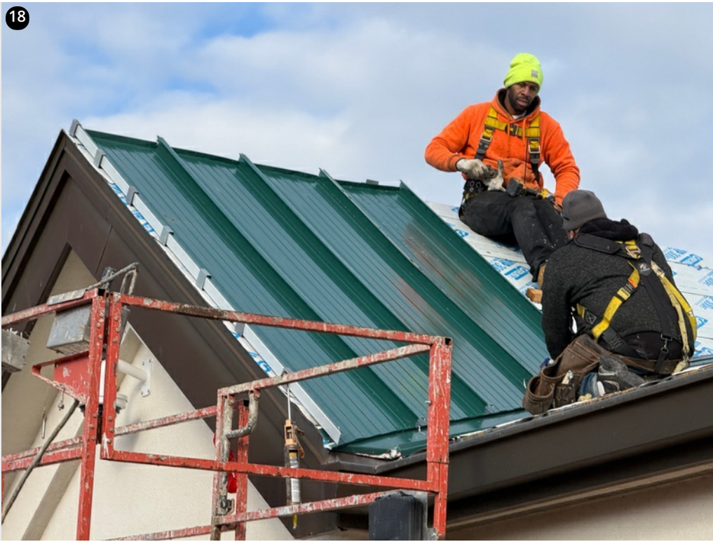
Crew installing panels on dormer- 11/29/24
