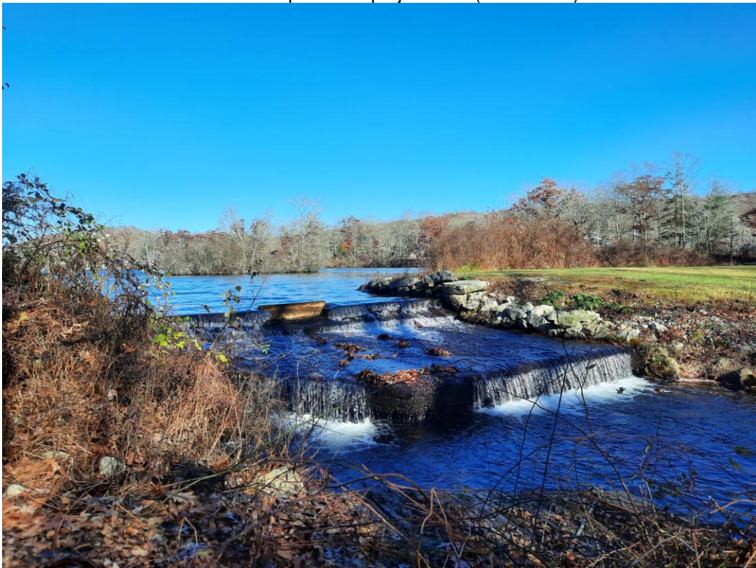
Looking north at Long Pond and Long Pond spillway (11/20/2023).
