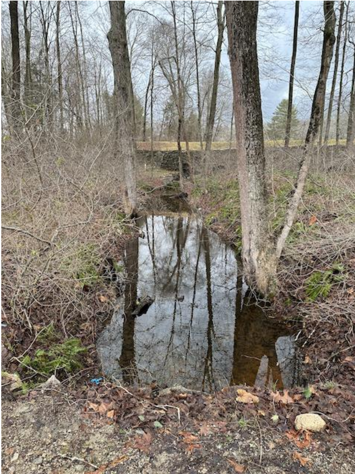
Photo #3 - Hyde Mill Pentway Road looking North
