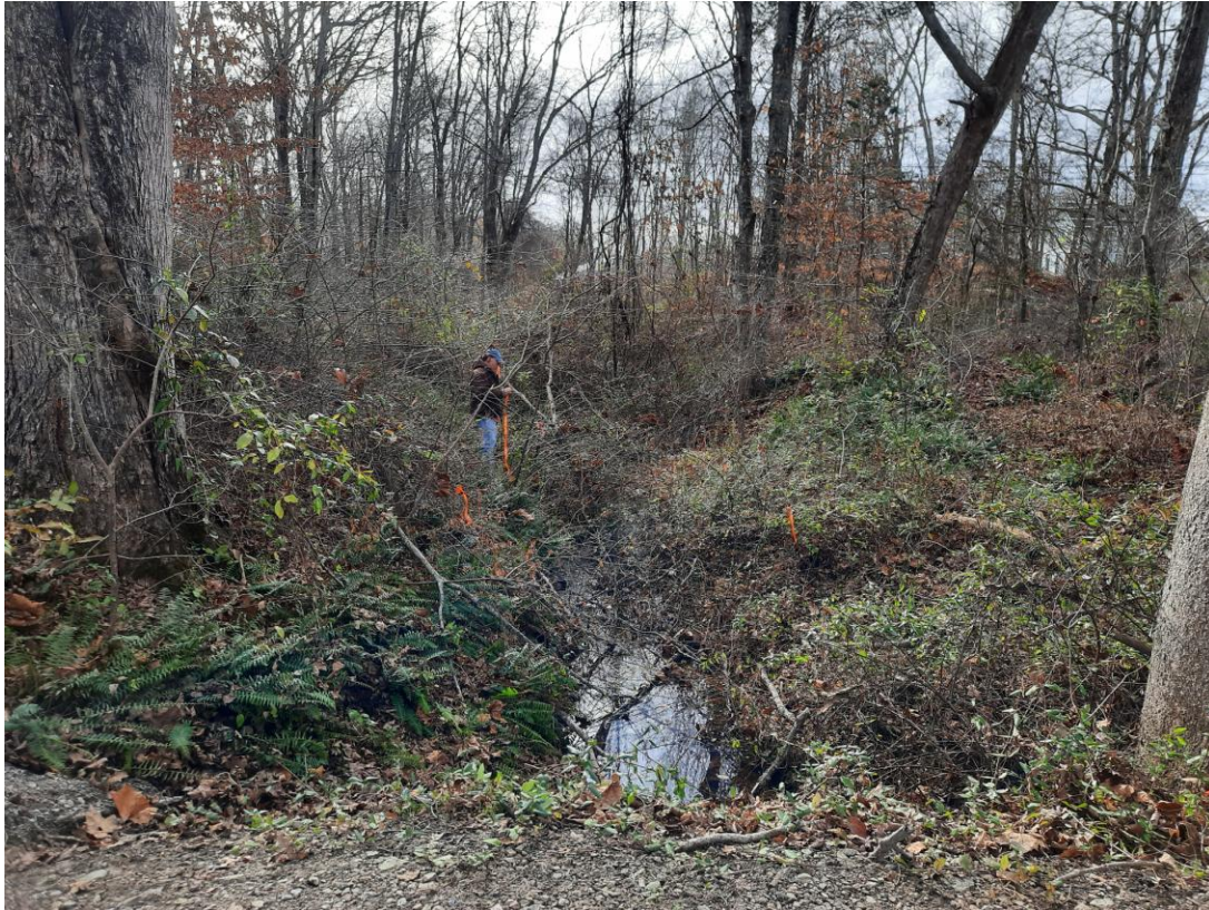
Looking south at narrow low flow channel south of Hyde Mill Pentway Crossing (11/21/2023).
