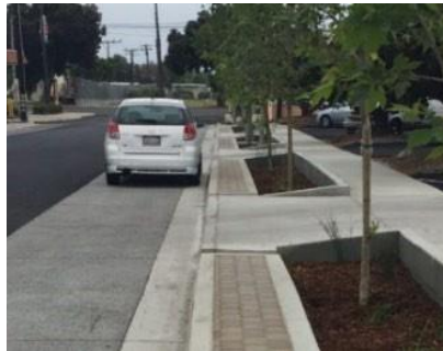
Figure 25: Permeable paving is used for parking. The sidewalk is defined by a permeable paved edge, planters for trees, and a change in surface from the sidewalk to the parking area.
