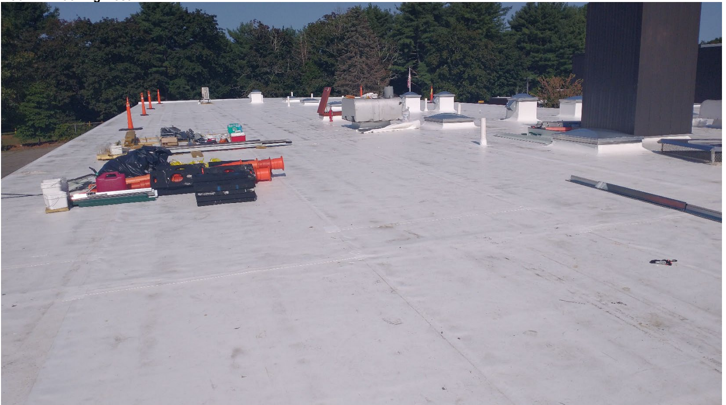
Roof A – Looking west
