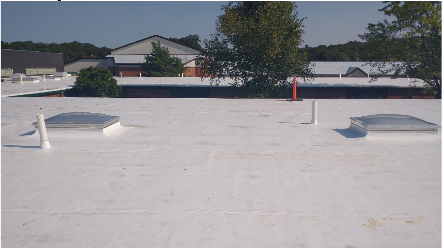
Roof A – Looking north
