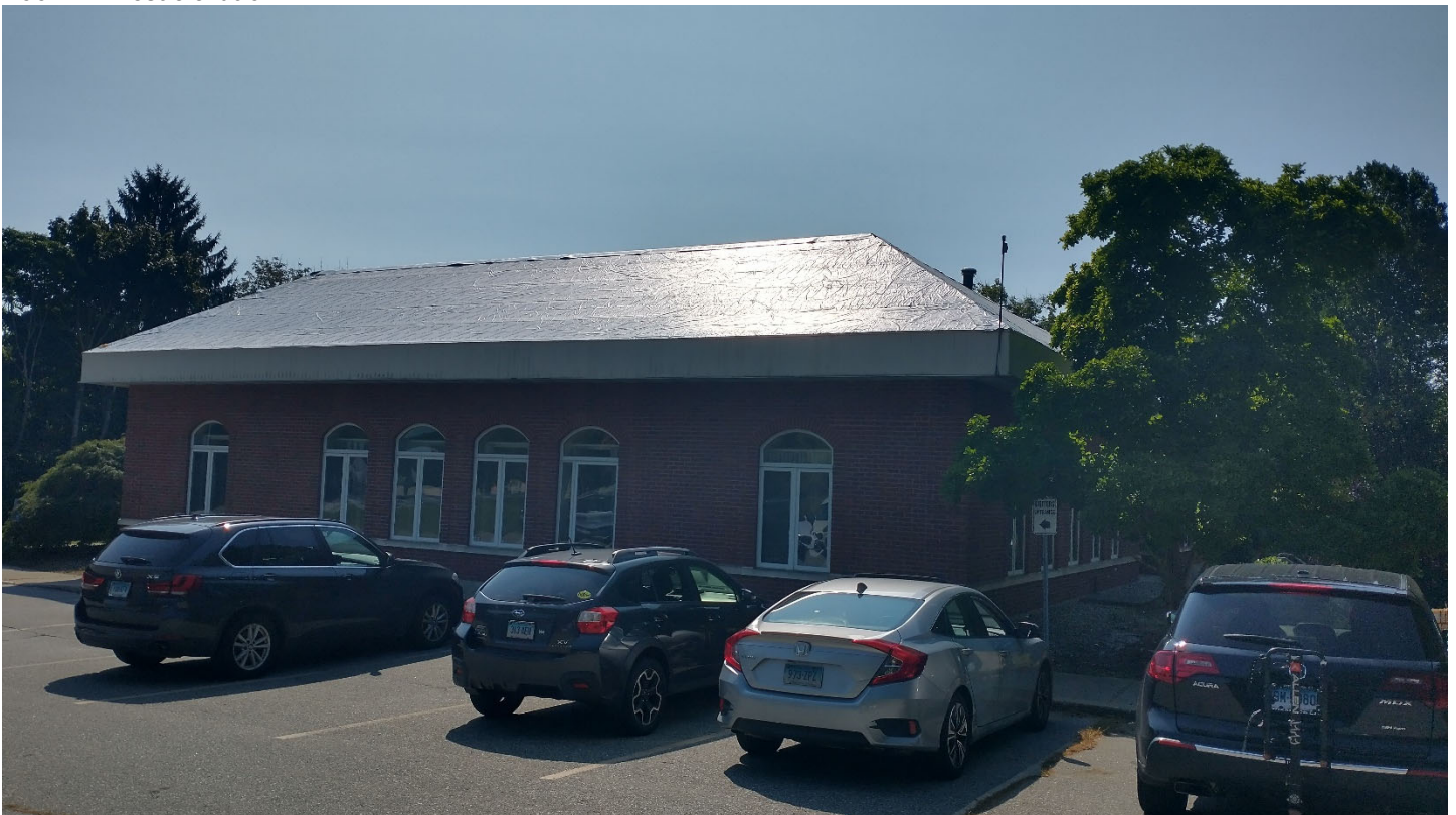
Roof A – West elevation
