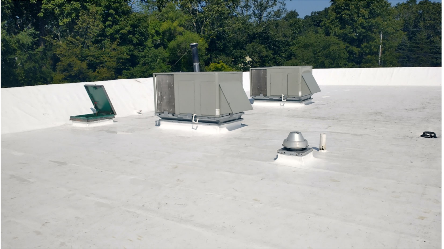
Roof B – Northwest view
