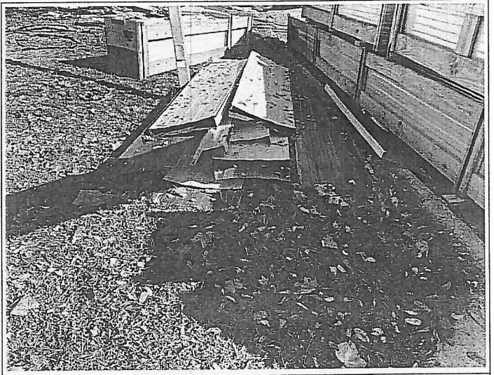
26. Sent by Wayne Donaldson. Scrap panels to be used in small cut conditions must be stacked and secured to maintain panel and rib shape.
