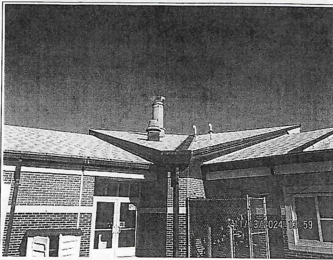
19. Curb flashings and pipe penetration boots will be installed according to the approved shop drawings and supplemental installation guide.
