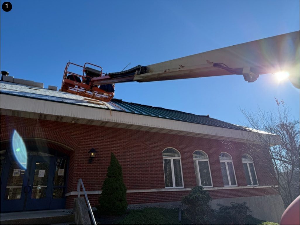
Crew installing panels on West side- 11/25/24
