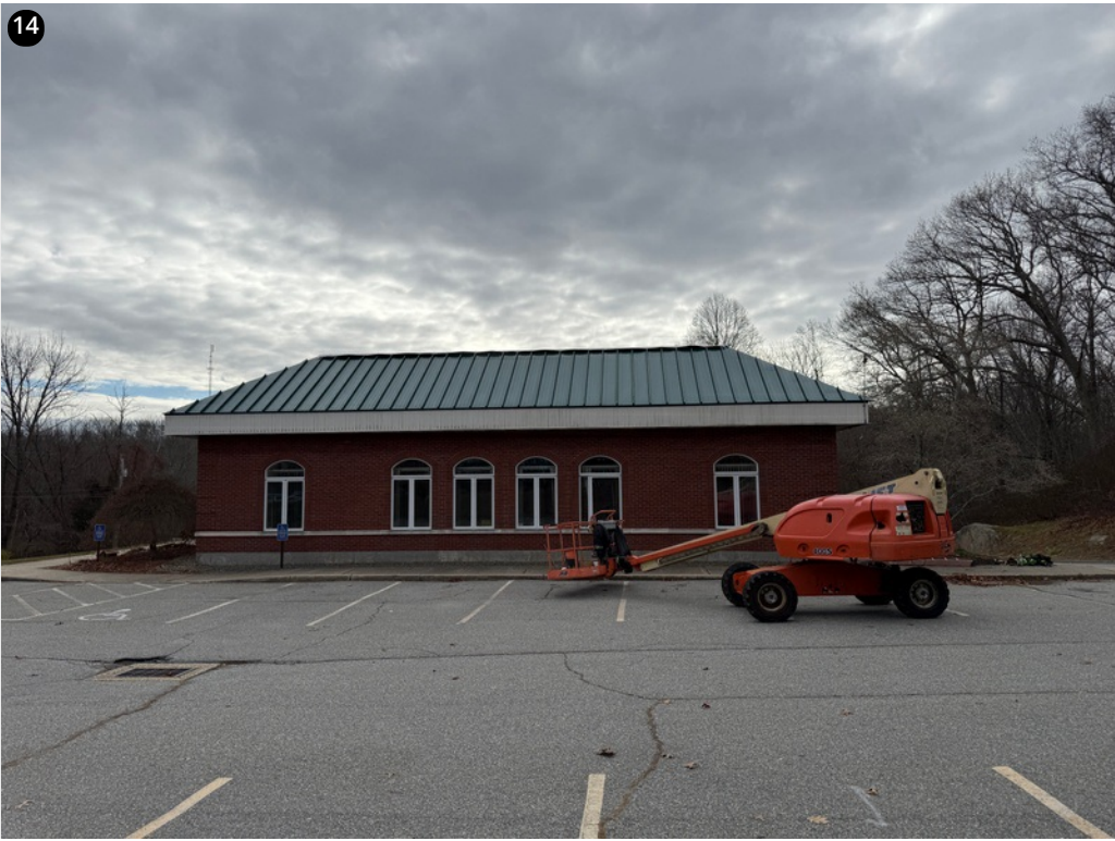
Overview- North side completed
