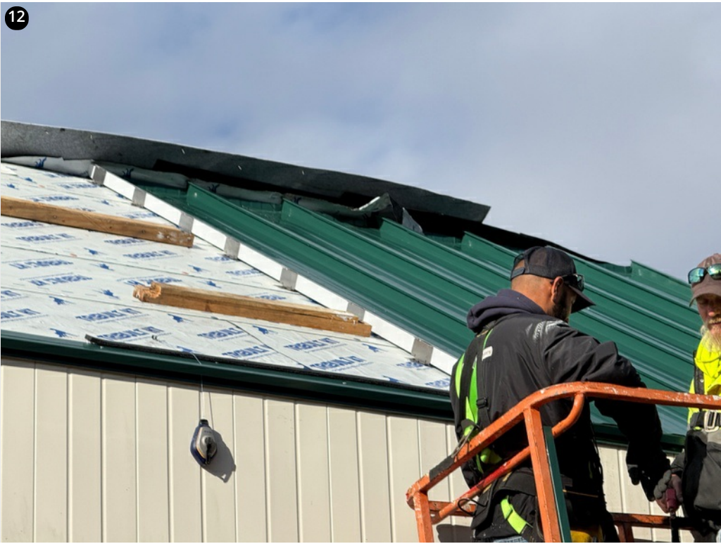
Crew riveting panel ends- 11/29/24
