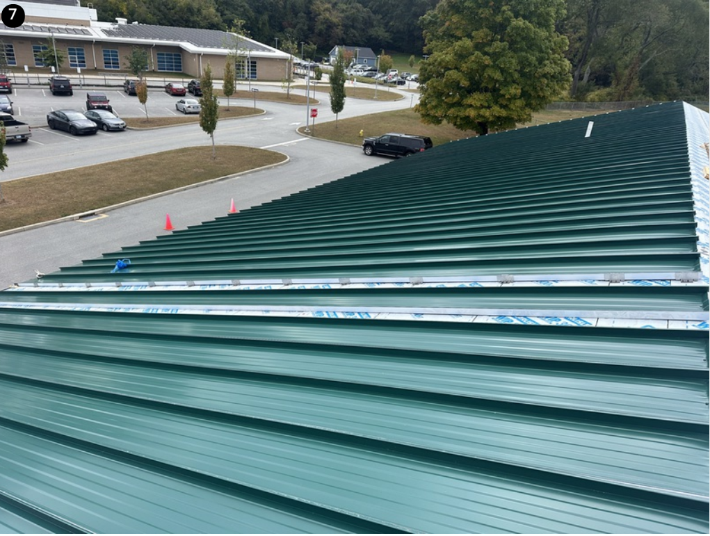
Overview- Installed panels
