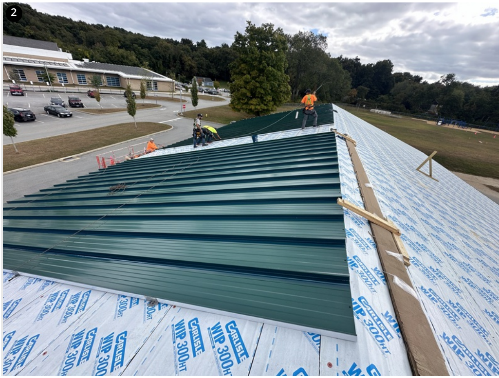
Crew fastening clips on field area
