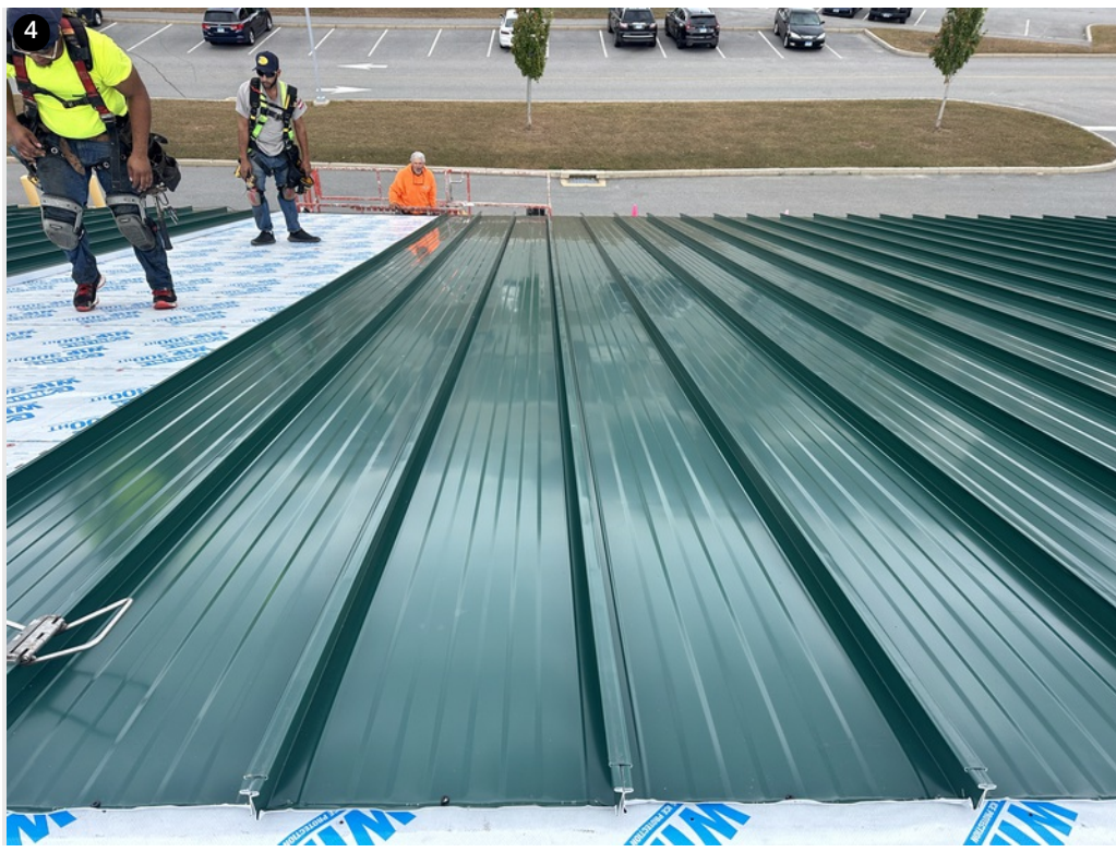
Installed panels- No oil canning
