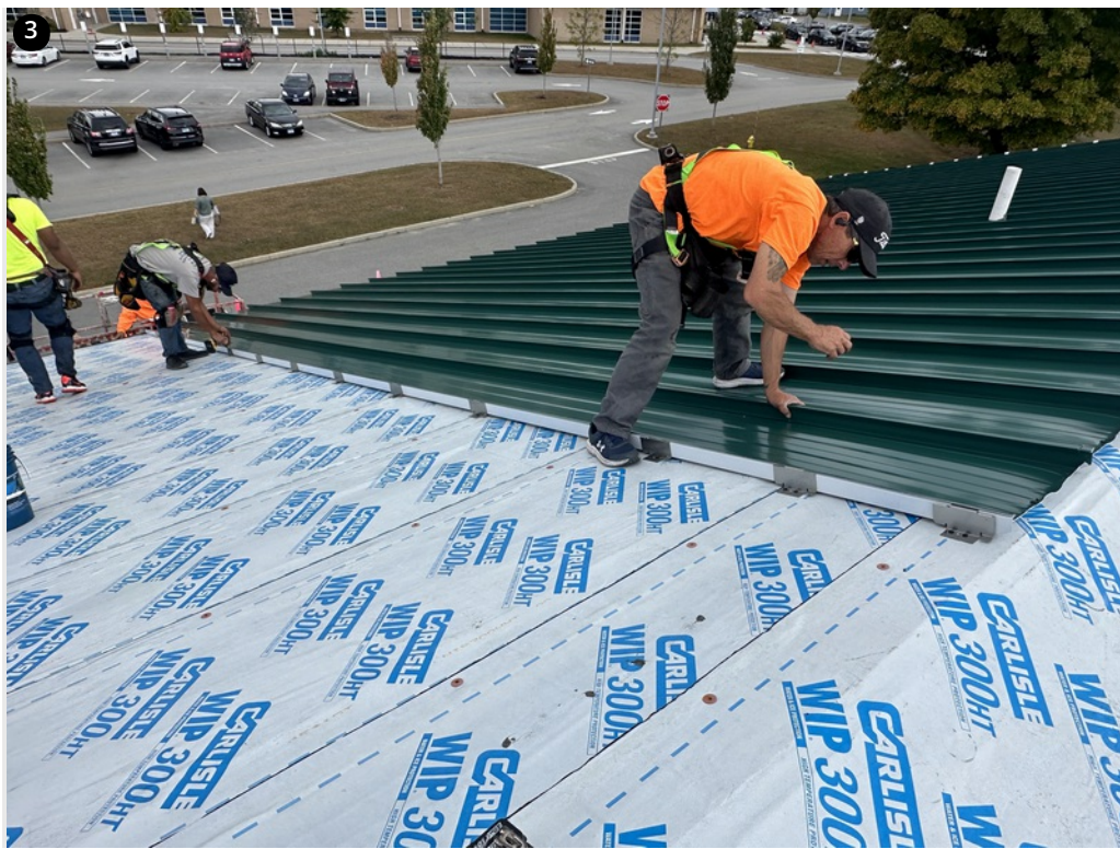
Field area- Clips spaced at 2'4" per spec
