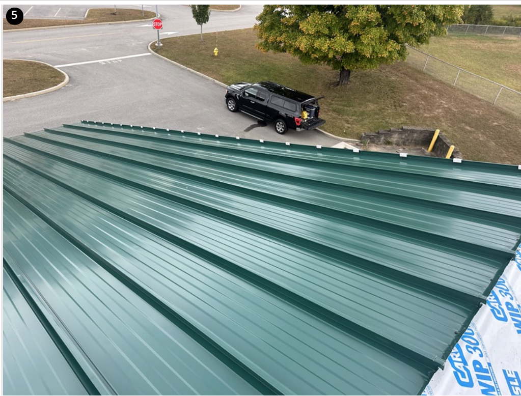
5 Perimeter edge zone- Clips spaced at 1'5" per spec
