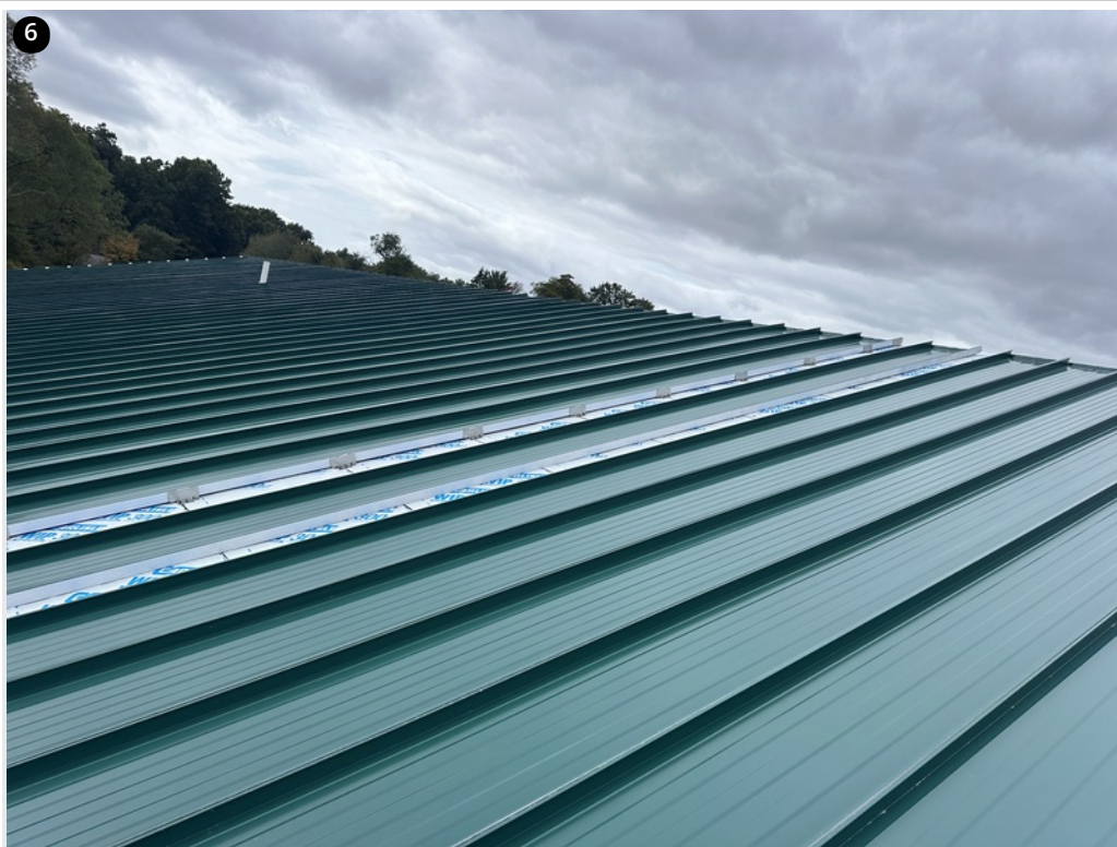
6 Field zone- Clips spaced at 2'4" per spec
