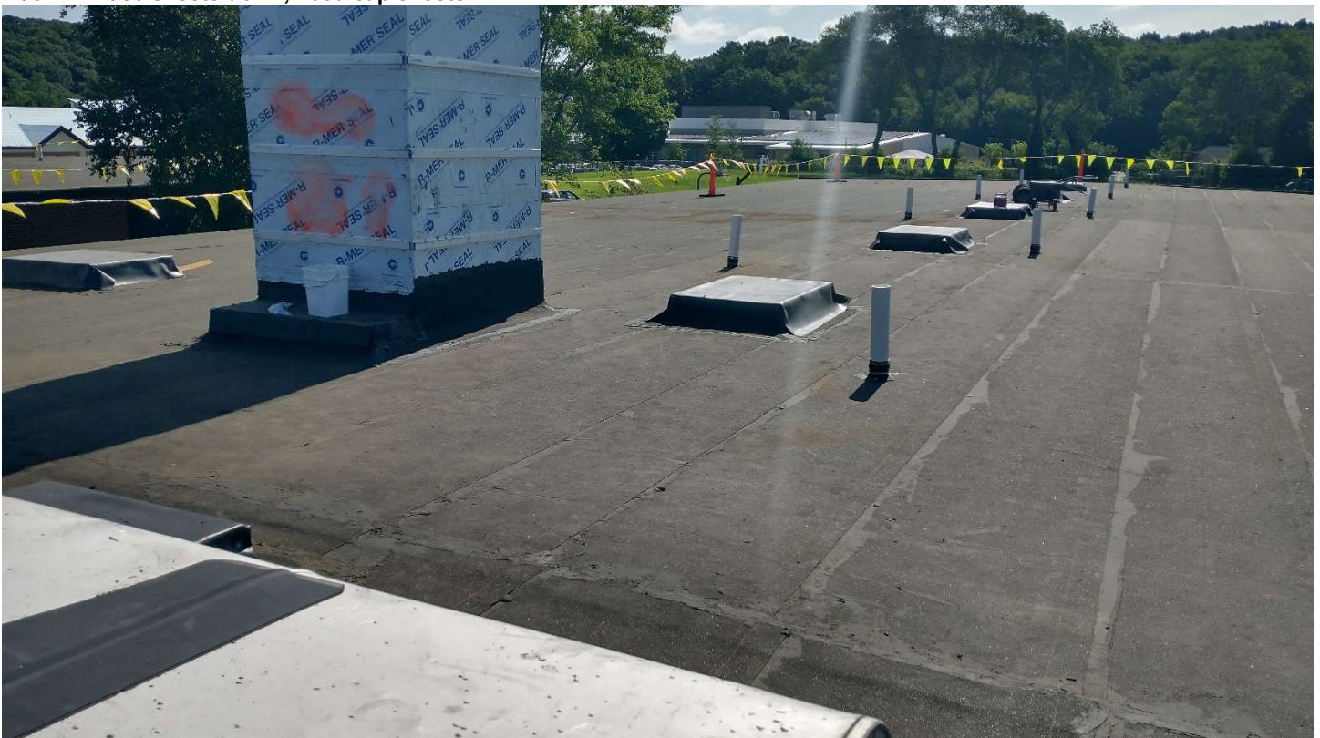
Roof A - Base sheets down, need cap sheets
