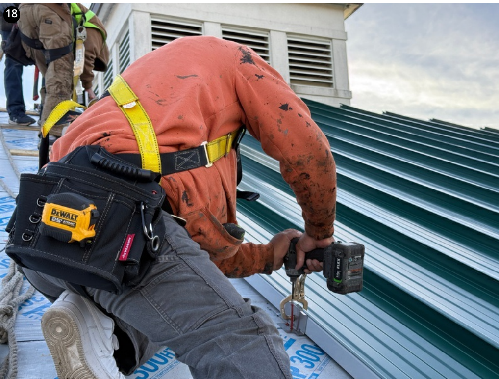
Crew fastening clips using red 8" fasteners
