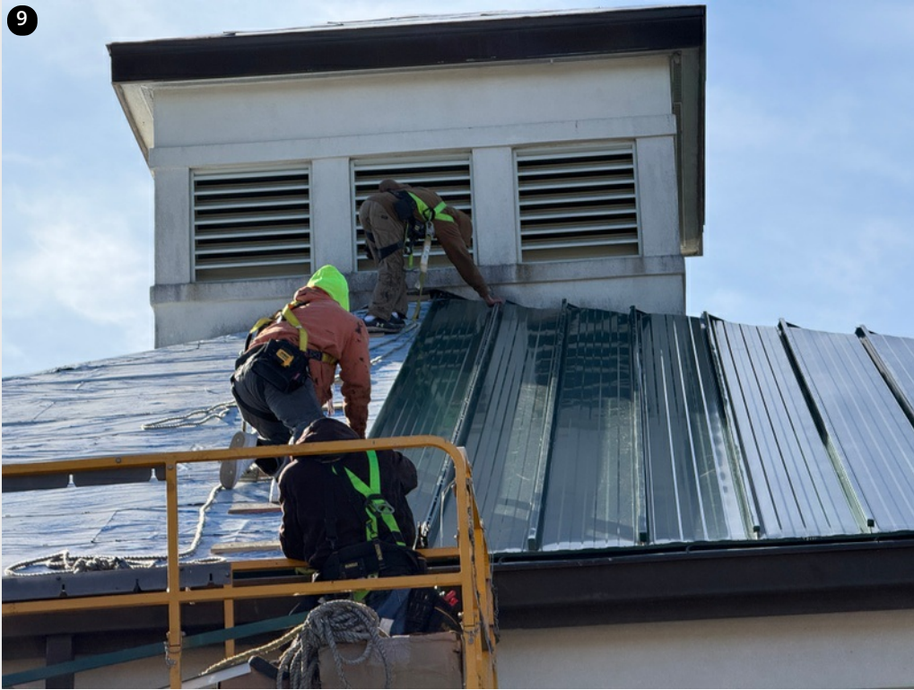
Crew installing panels and securing to fastened clips- 11/14/24
