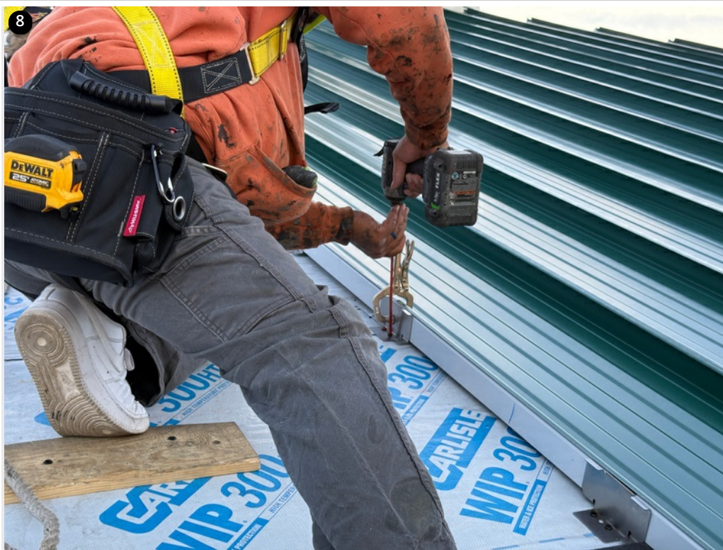
8 Crew fastening clips spaced at 1'8" using 8" red fasteners- 11/14/24
