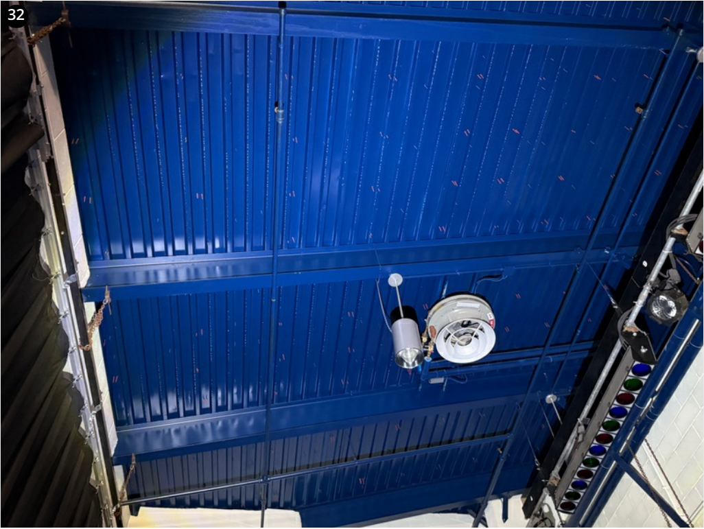
11/18/24- Fasteners observed properly penetrating deck
