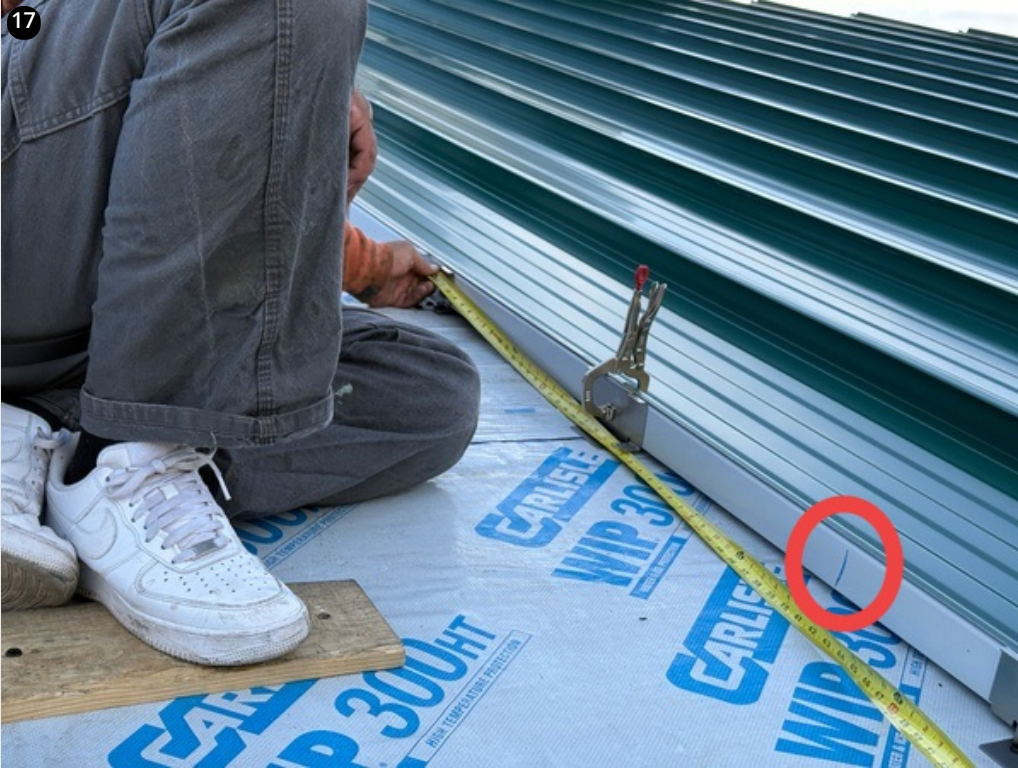
Clips spaced at 1'8" according to zone
