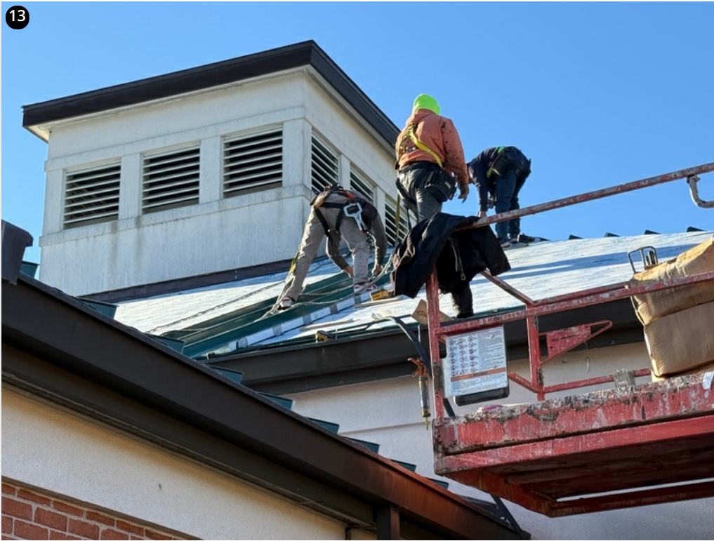
Crew fastening clips using 8" red fasteners- 11/15/24
