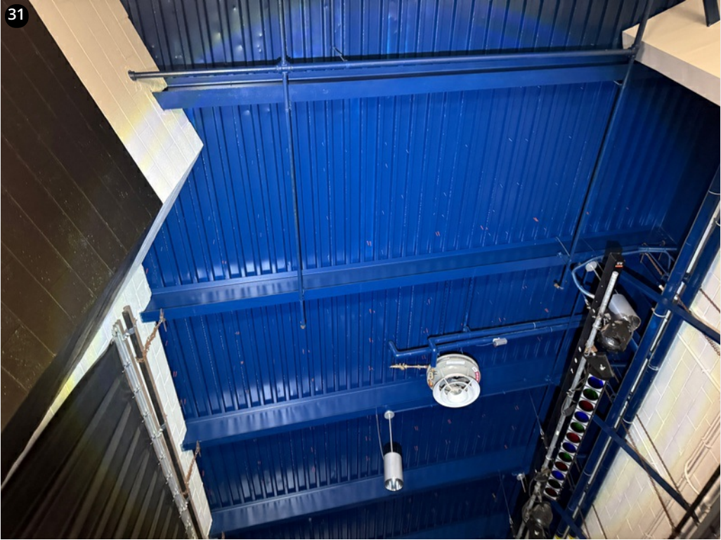
11/18/24- Fasteners visible properly penetrating deck
