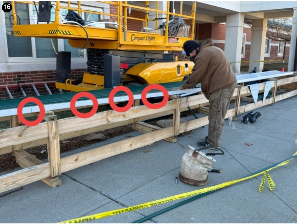
Crew marking out clip spacing per zone on panels prior to install- 11/15/24
