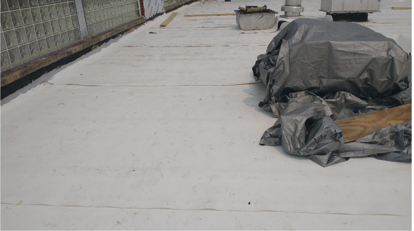
Roof A – Seams need to be welded
