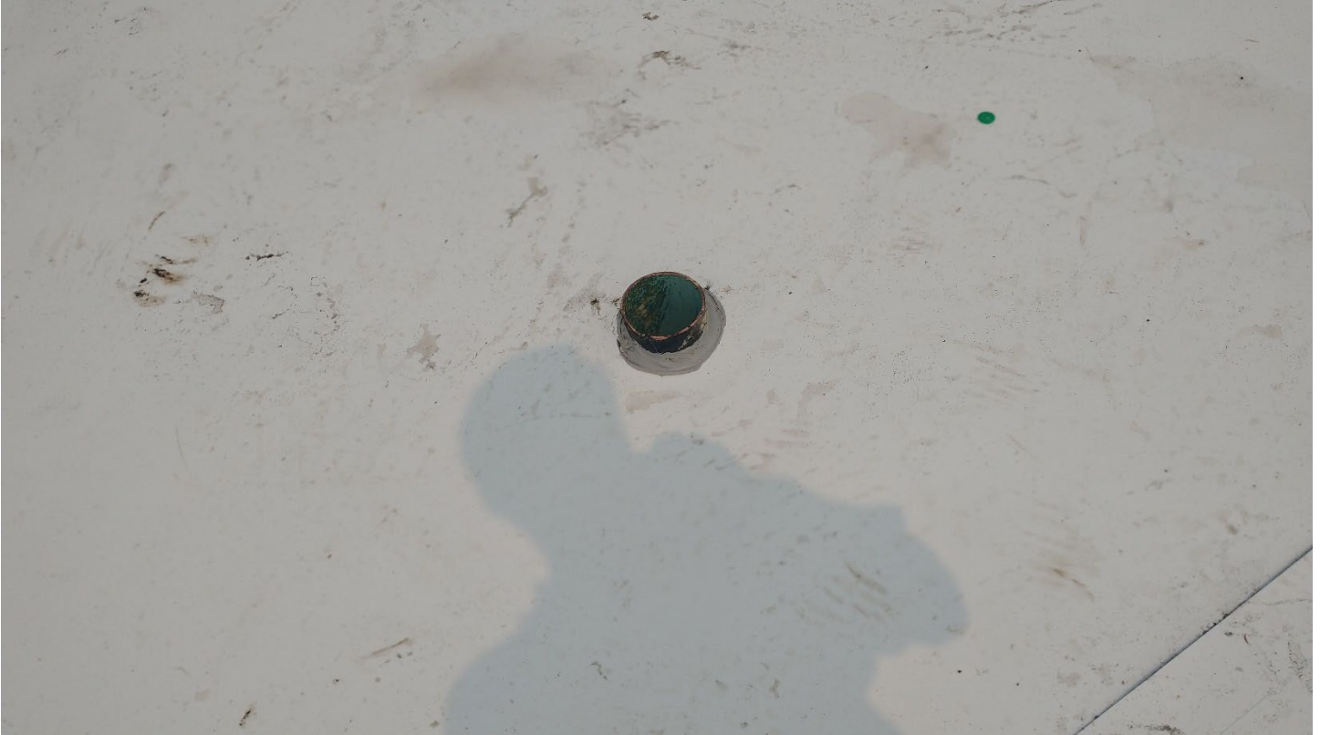
Roof A – Roof vent sides are too short will insert an inner coupling to hold the top vent pipe to the lower
