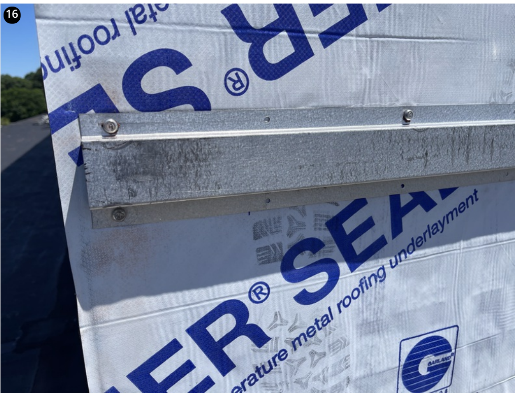
Hat channels for wall panels installed properly
