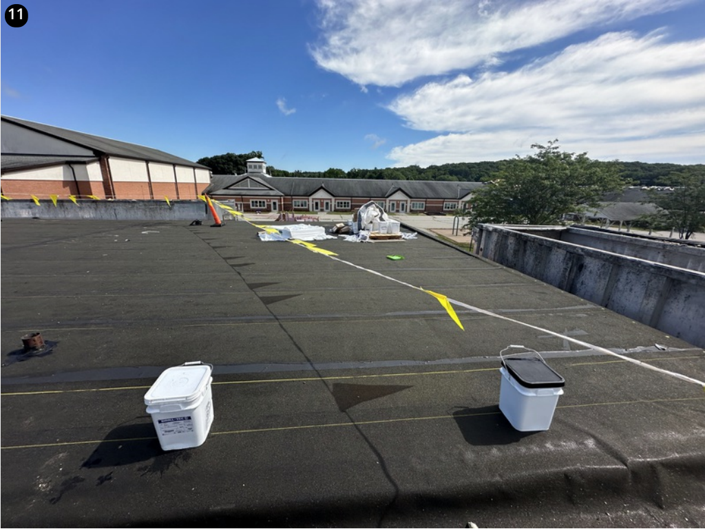
Night tie-ins complete and weighted
