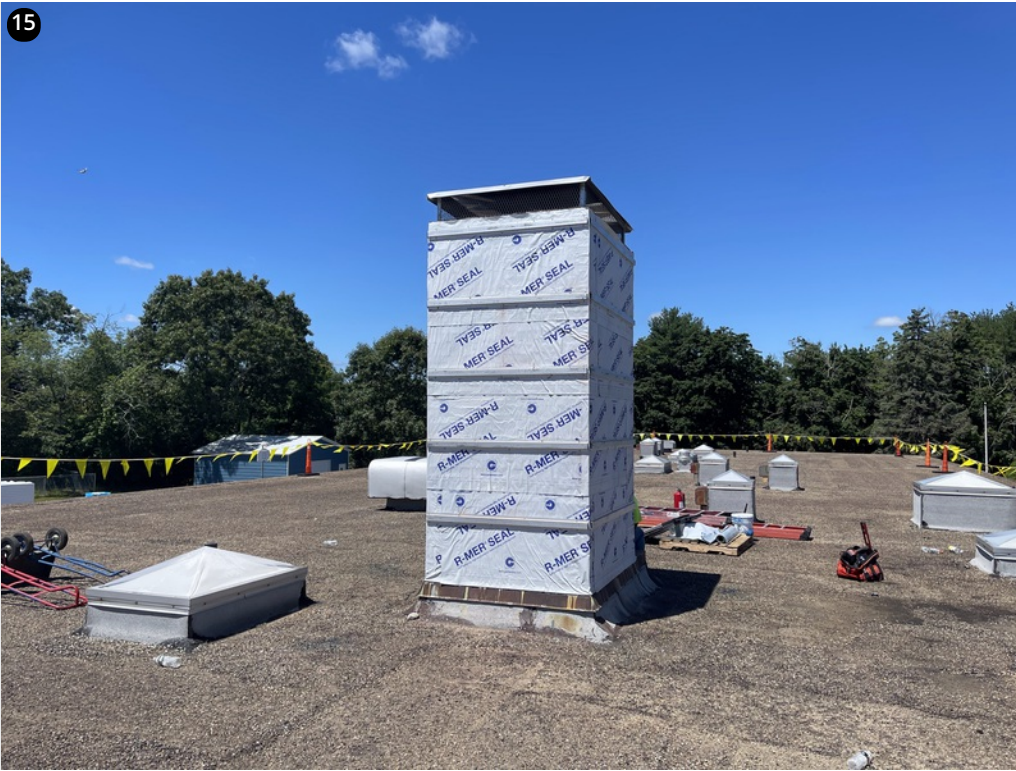
Chimney primed, wrapped and hat channeled
