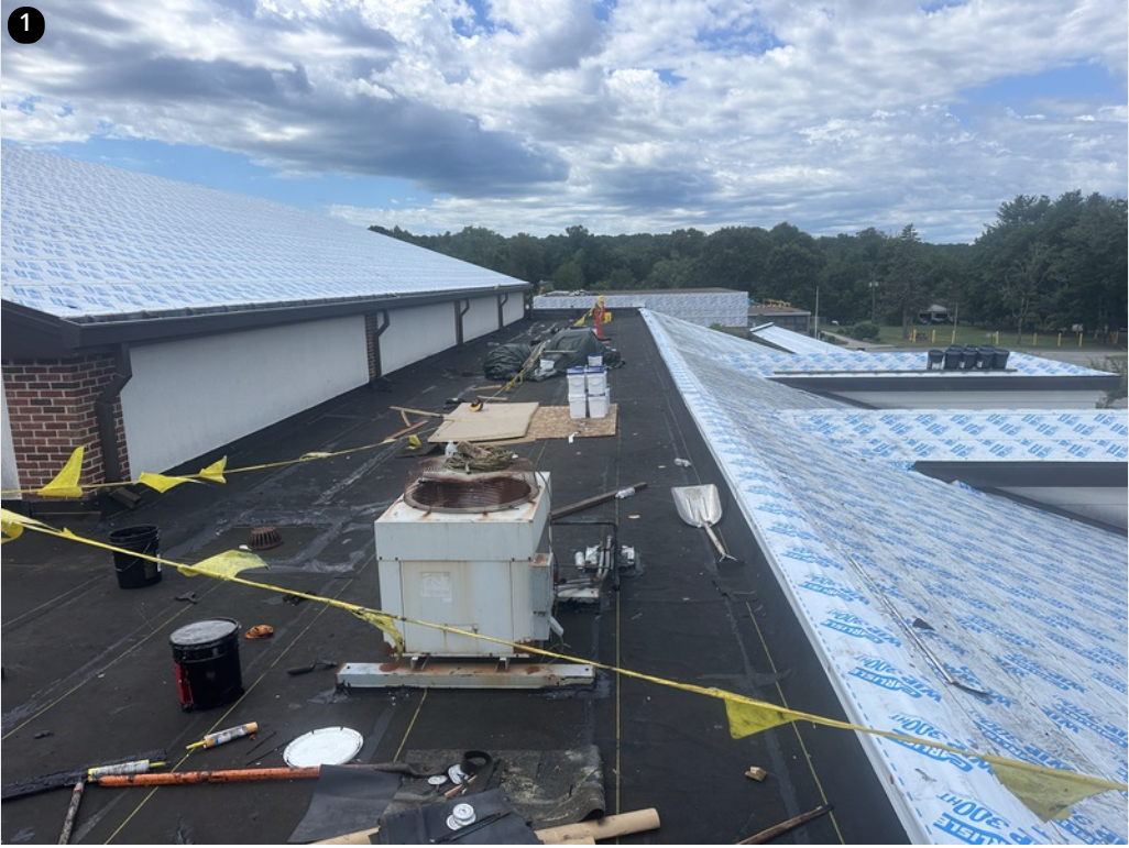
1 Overview- Completed base sheets on low slope area
