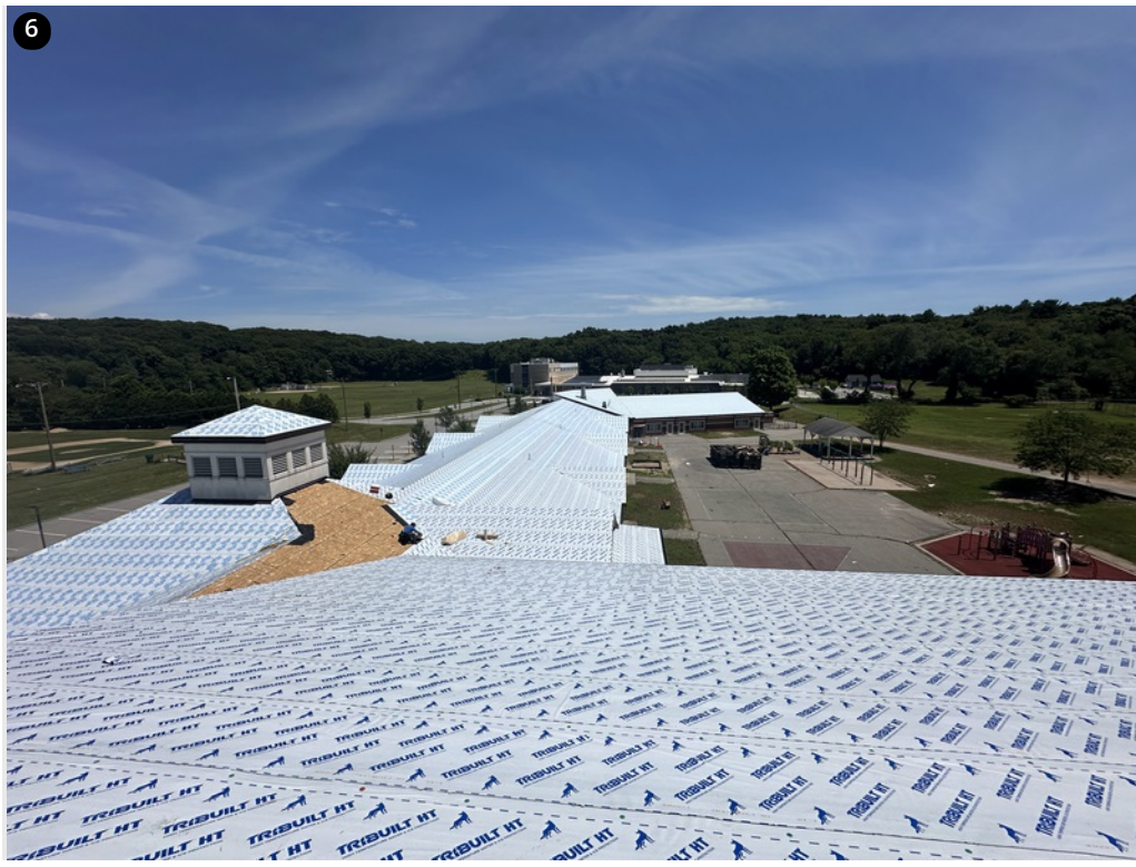
Overview- 99% completed ice and water installation
