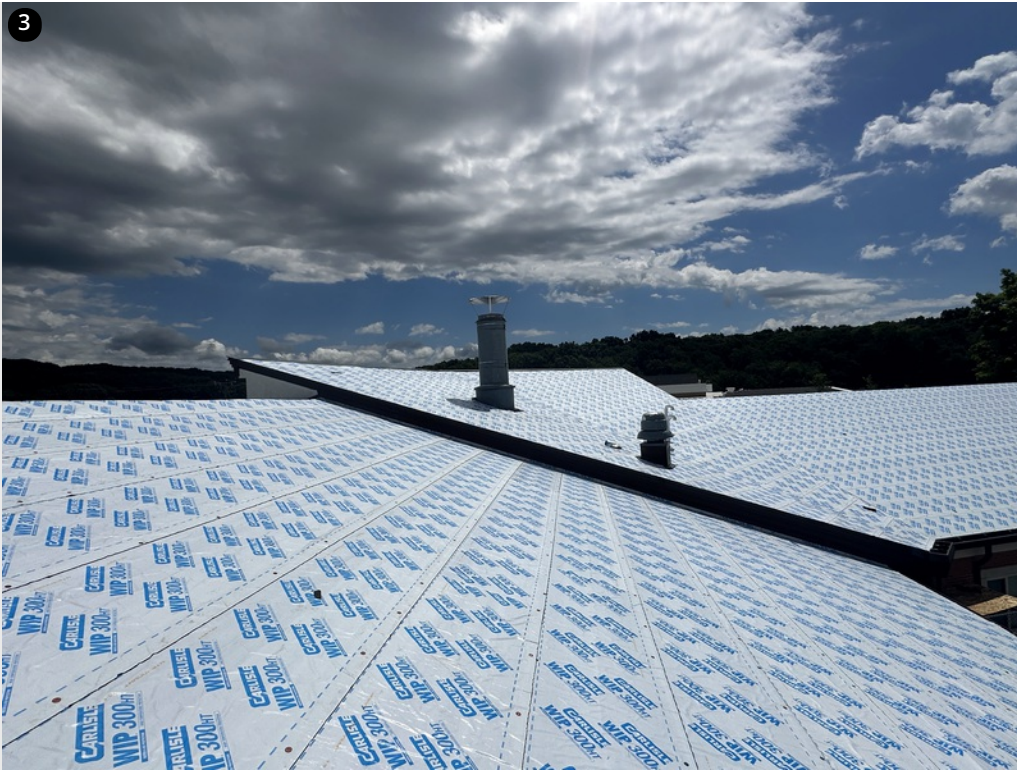
Overview- Completed ice and water layer on sloped sections
