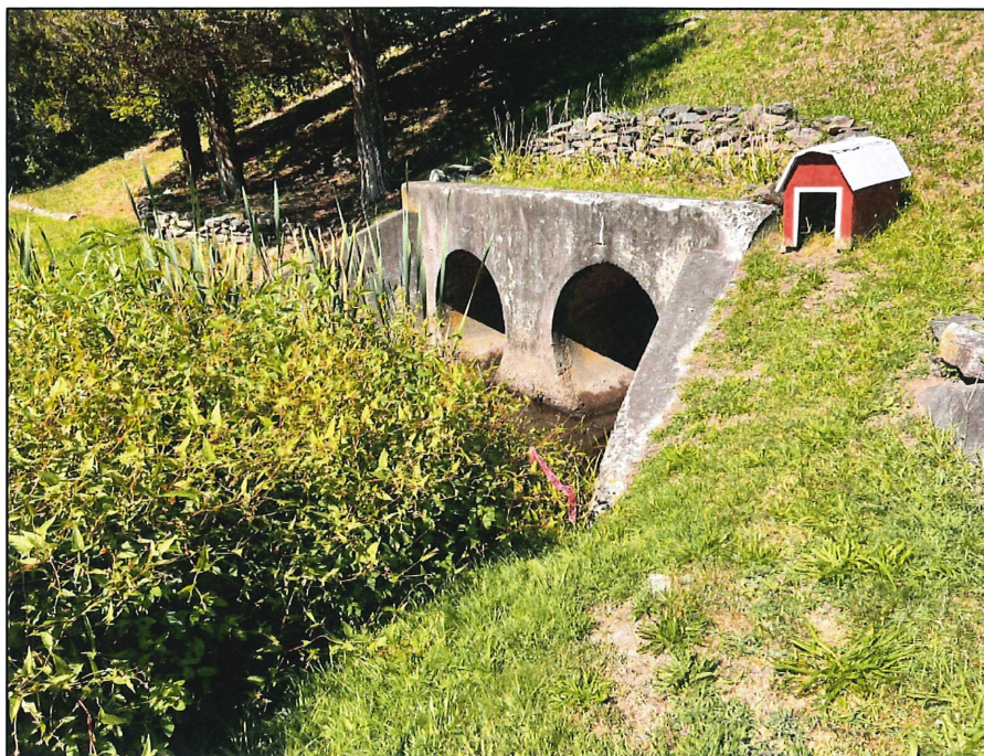
Photo 3: View of inlet at Route 12.
