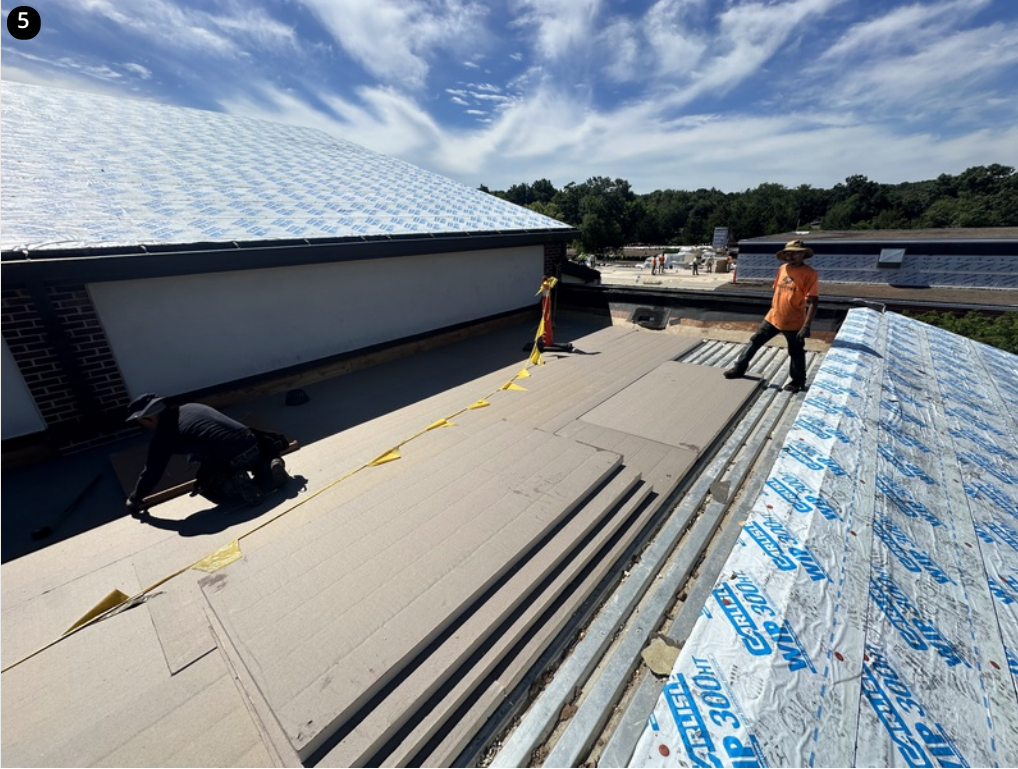
EPDM section ripped to metal deck- Crew laying out insulation boards
