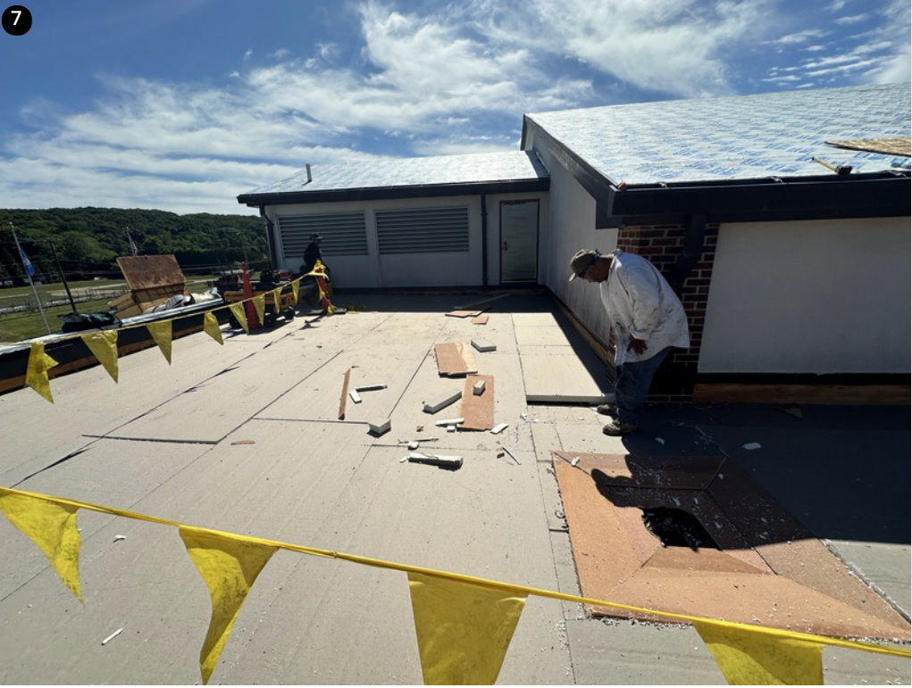
7 Insulation laid out on ripped EPDM section
