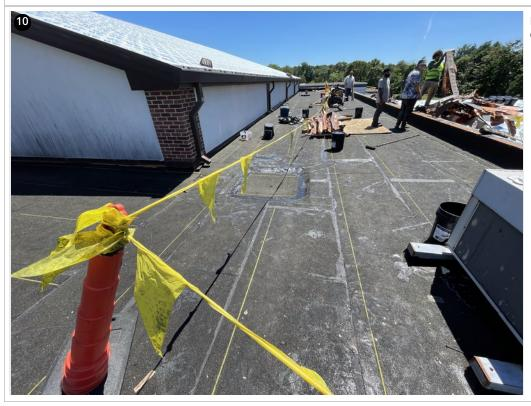
Low slope roof section base sheet is completed and drains are temped in
