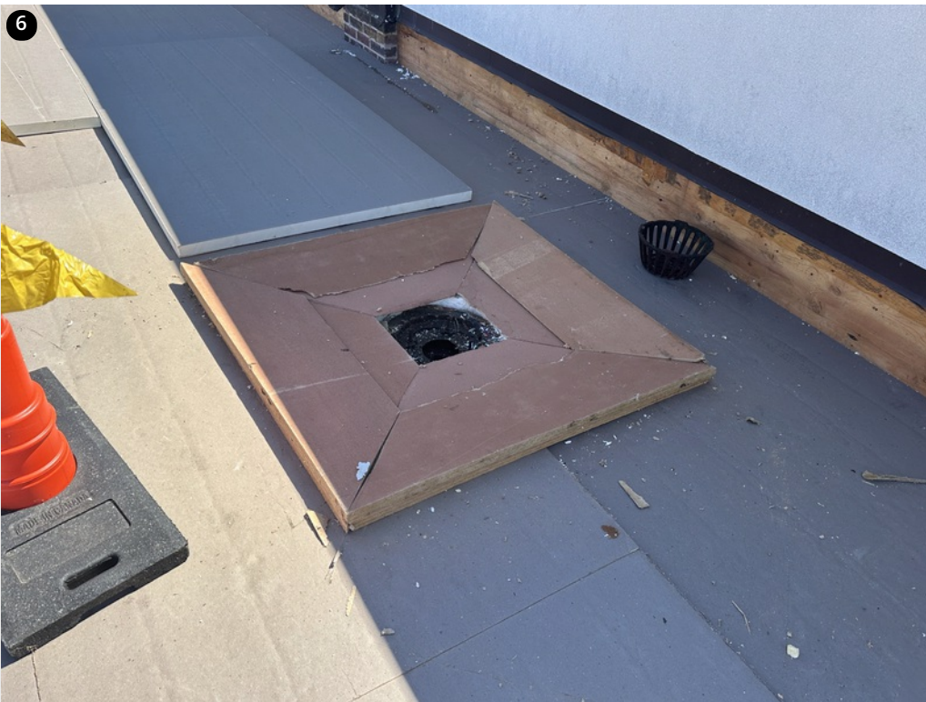
Drain sump built up with insulation
