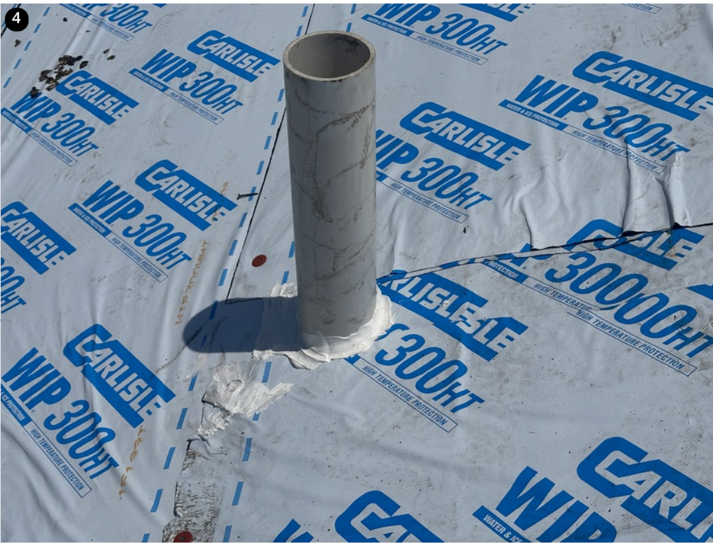
All penetrations tied into ice and water layer using proper sealant
