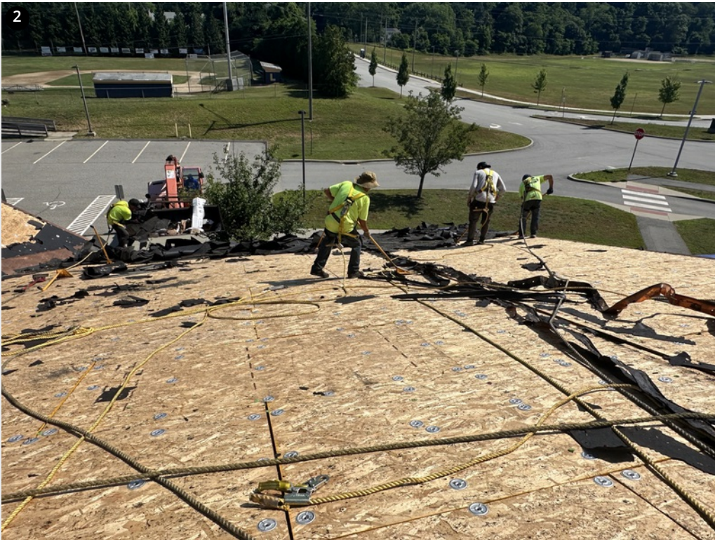
All crew following proper safety precautions- Harnesses, tie offs etc
