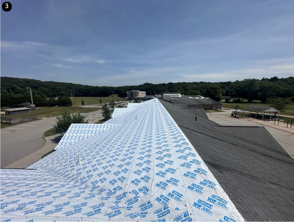
Ice and water layer installed on parking lot side
