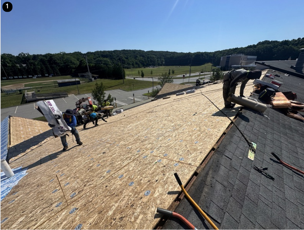
Crew ripping shingles on sloped section facing the baseball field
