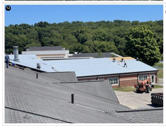
The shingle crew ripped the furthest interior section and finished the valley
