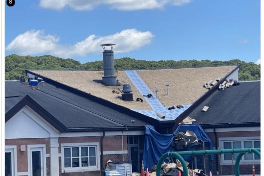
Valley section ripped to deck- Valley reinforced with ice and water layer
