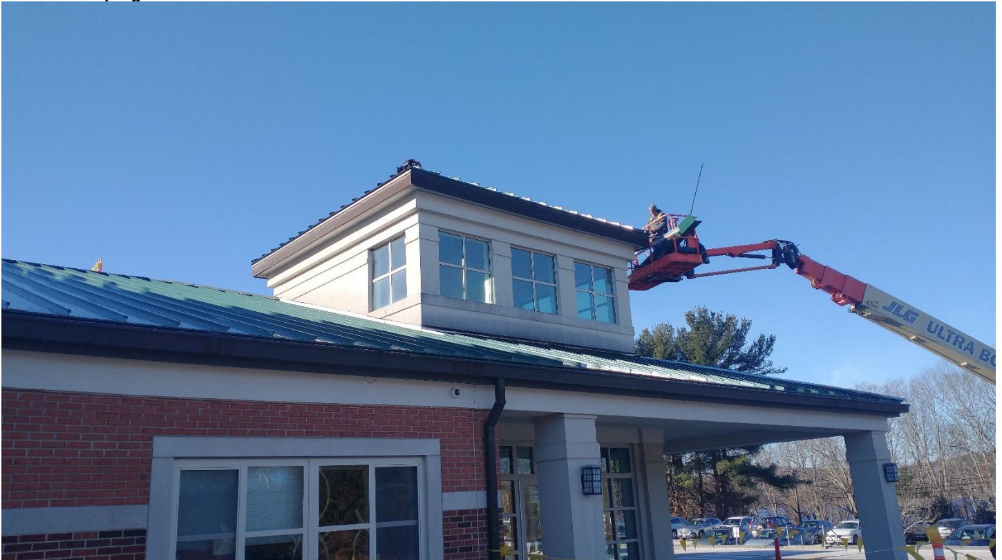
Trim work in progress on the “tower” of roof A
