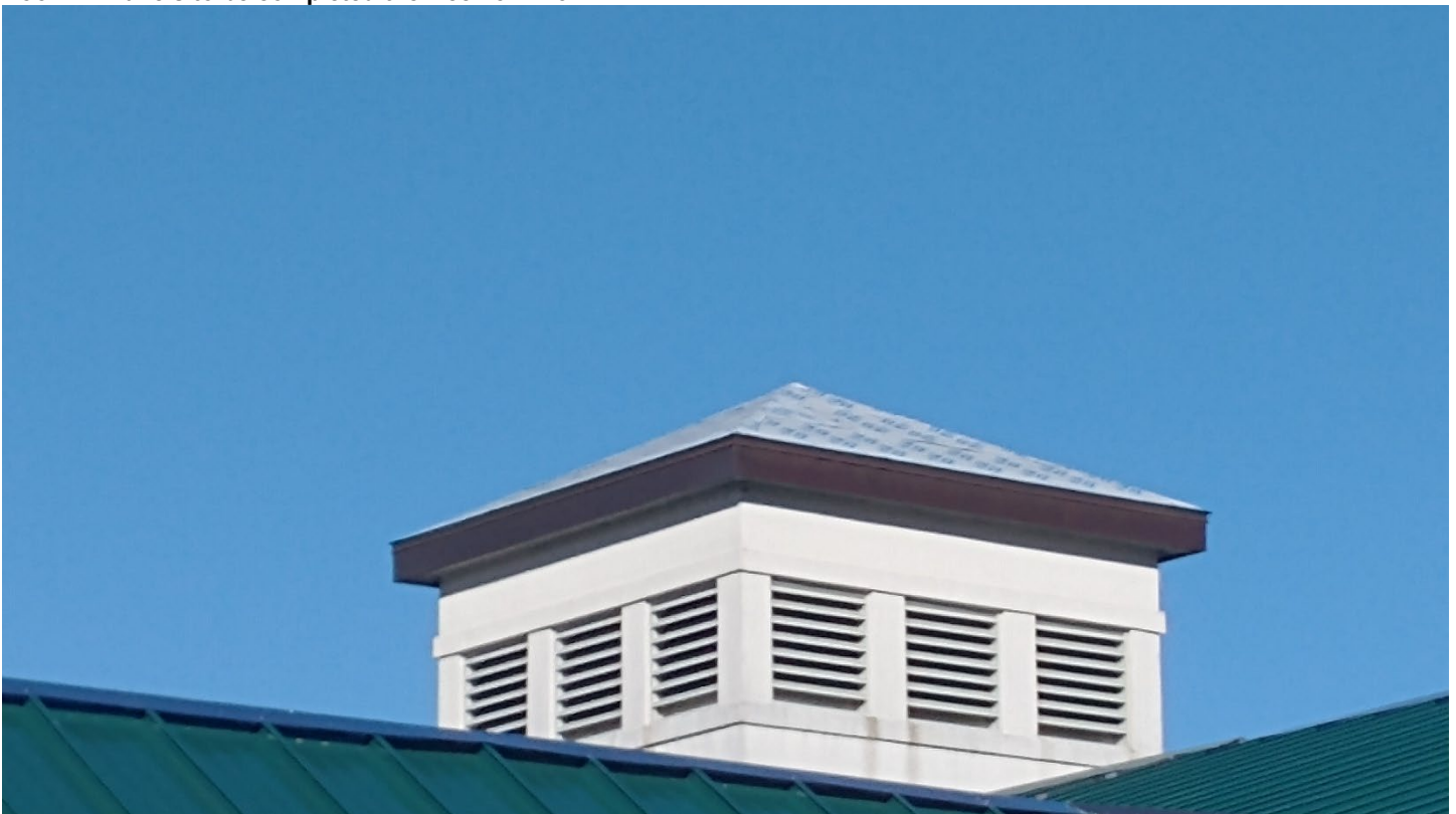
Roof A – Panels to be completed the week of 1/13 -17
