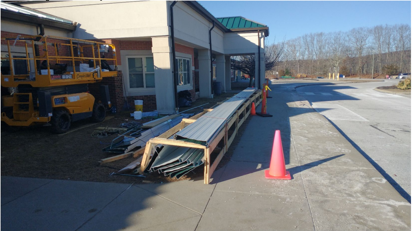
Area for storage of the workdays material.
