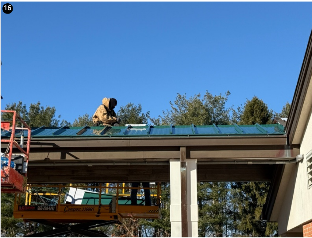
Panels being installed on walkway roof- 12/6/24
