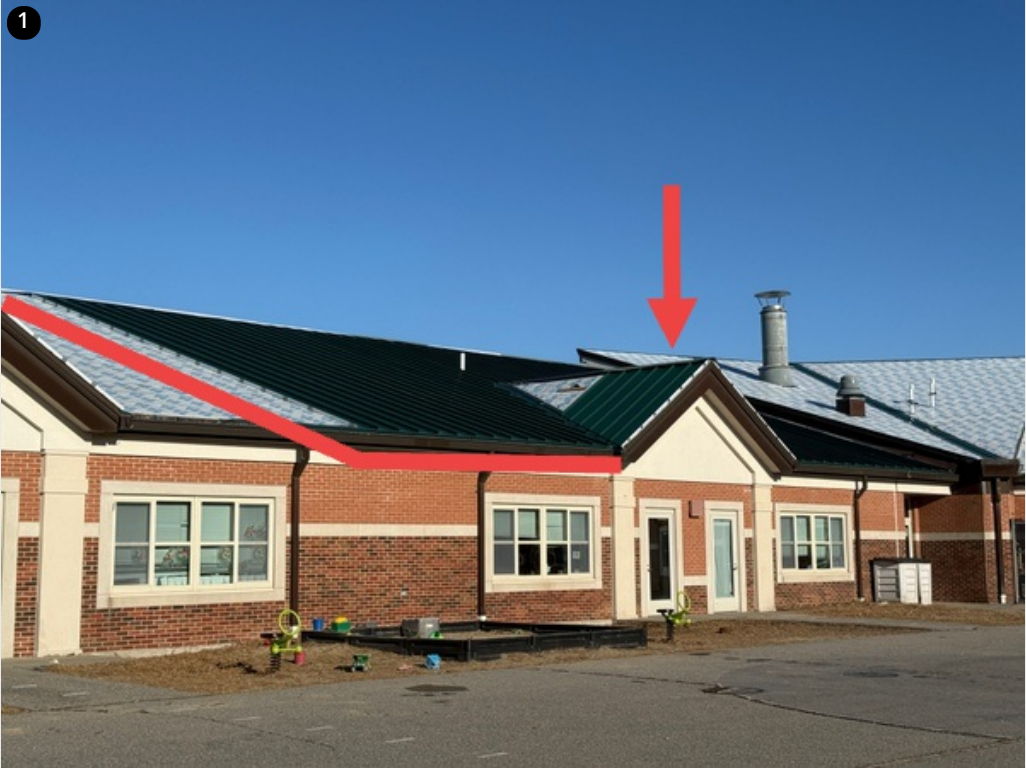
Panels installed on field areas and dormer- Saturday 11/30/24
