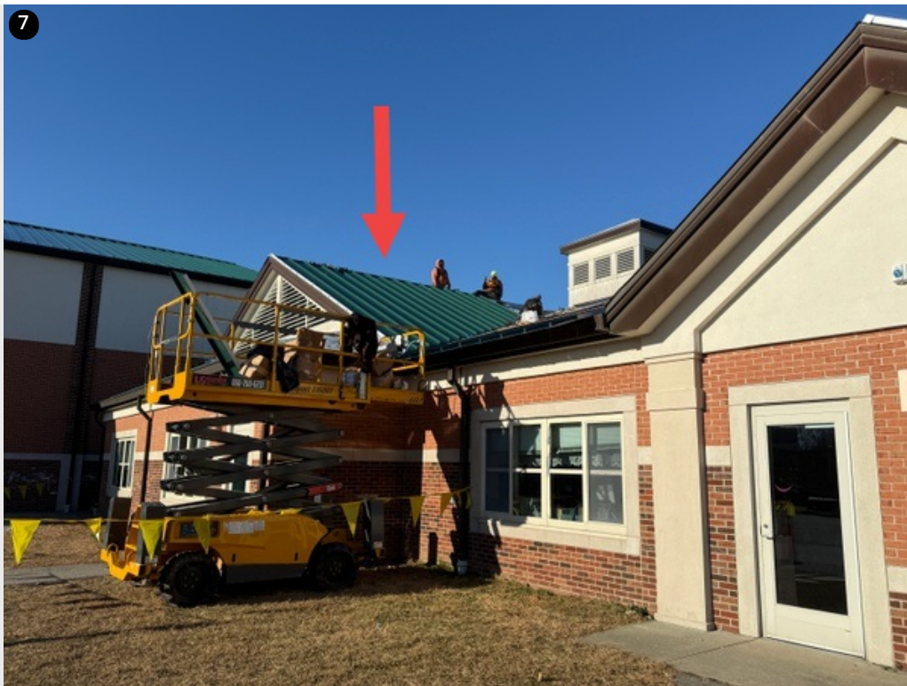
Crew installing panels on dormer- 12/2/24
