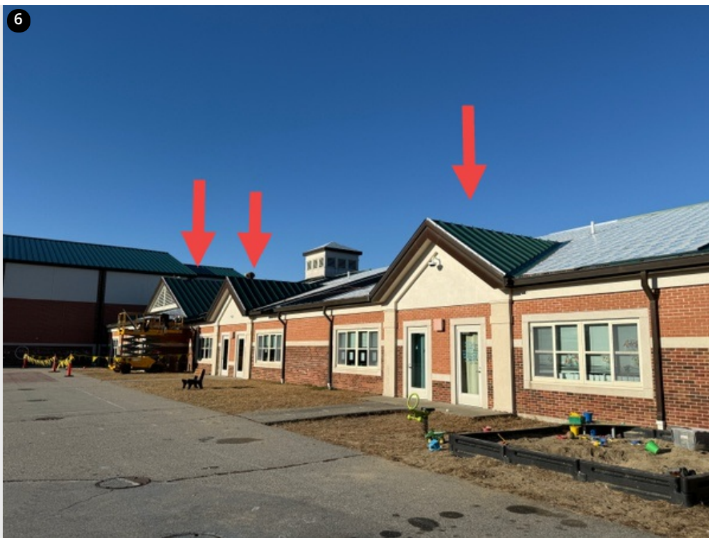
6 Panels installed on dormers- Saturday 11/30/24
