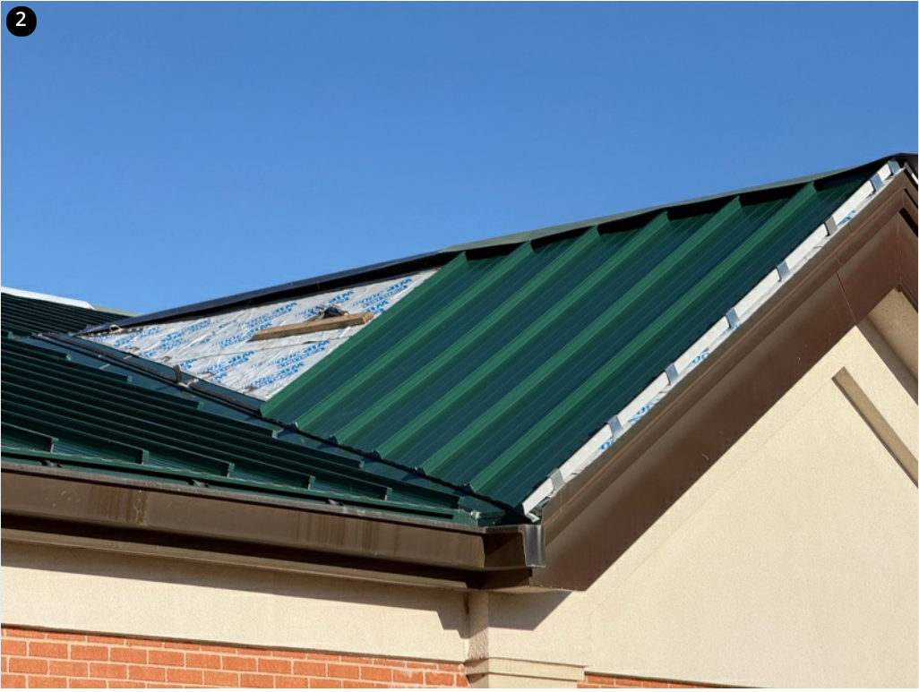
Panels installed on dormer- 11/30/24
