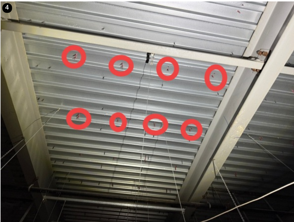
Fasteners observed properly penetrating roof deck- 11/30/24
