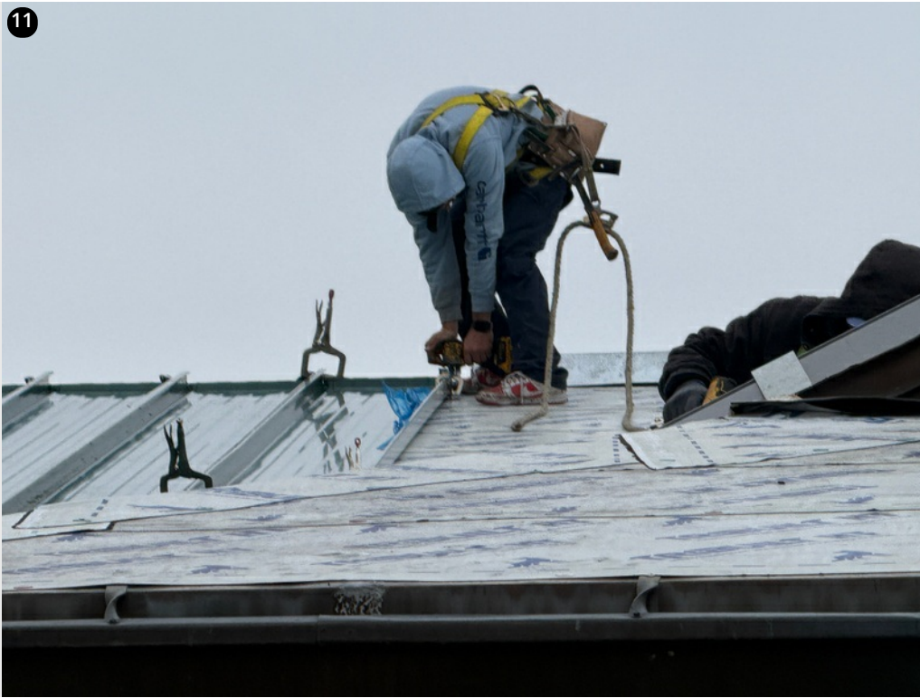
Crew fastening clips on field section behind copula- 12/4/24
