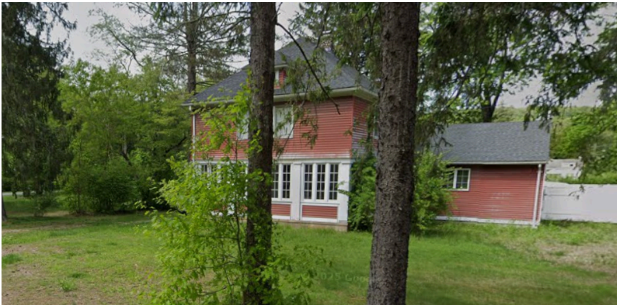
American Four Square - hipped-roof w pedimented fenestration and gabled additions- John J. Lawless House, 1912 (possible Sears Roebuck catalog design)
