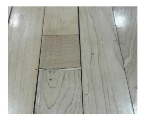
It is difficult to get a full sense of the "waviness" of the floor in some locations just from a 2D photo, but hopefully, the degree of cupping of the boards in this picture comes through.
