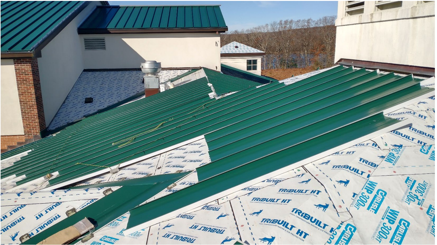
Roof A – Panels to be fastened in other areas
