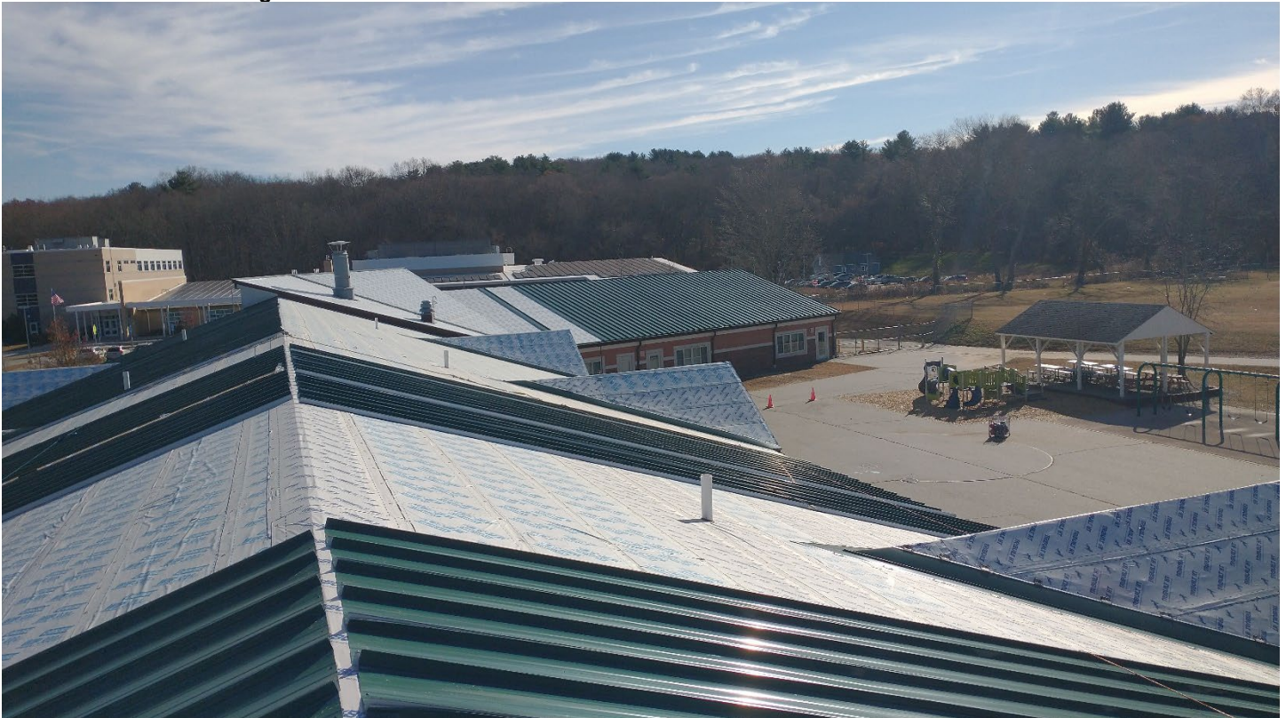
Roof A – Overview looking east
