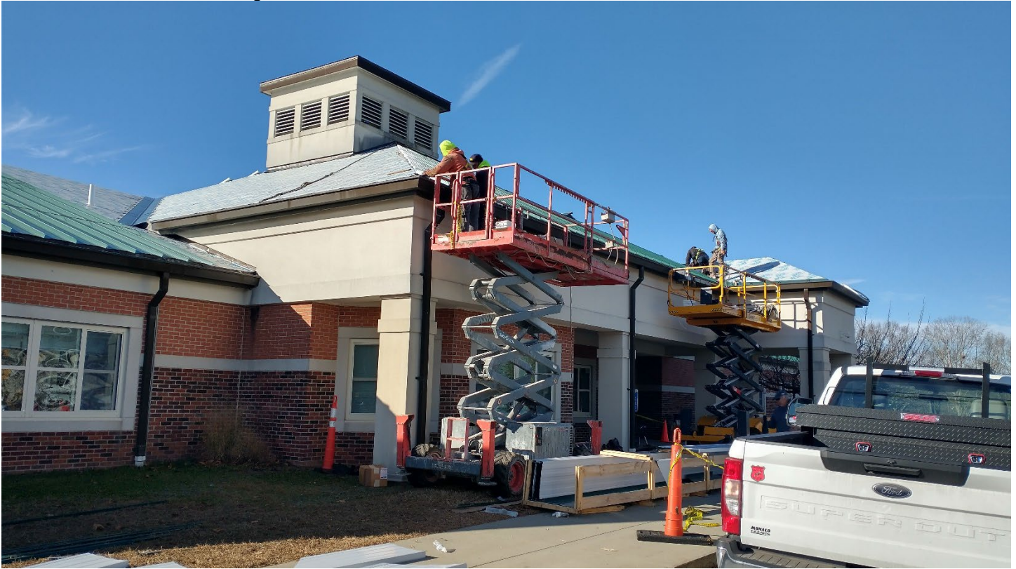
Roof A – North elevation looking southeast
