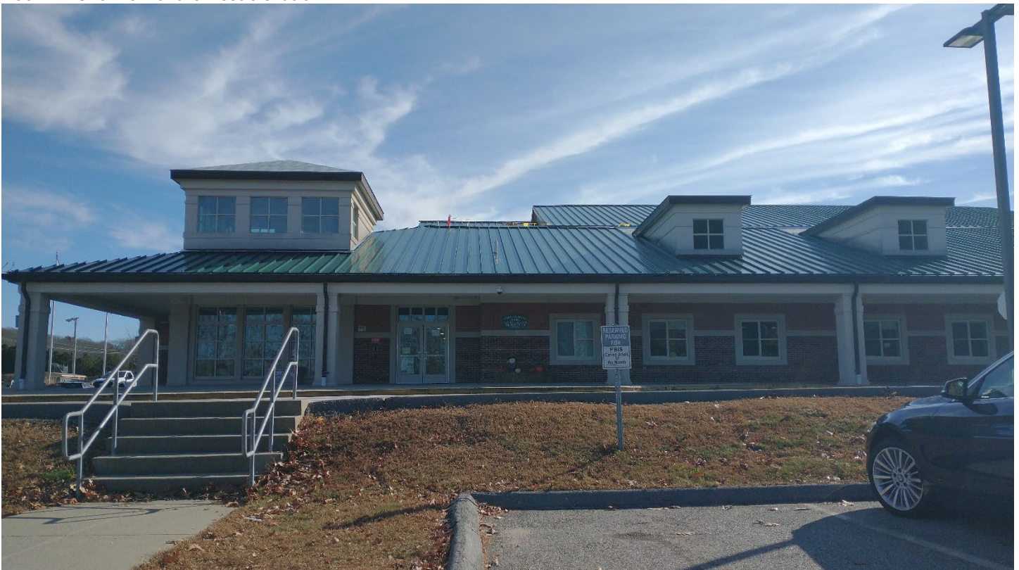
Roof A – Overview of the west elevation
