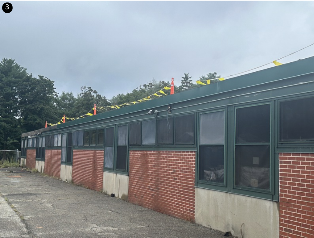
Fascia partially installed
