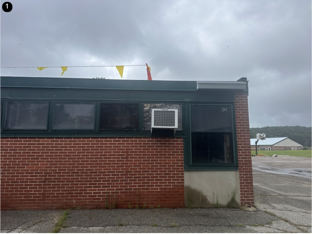
Fascia and gutter sample installed
