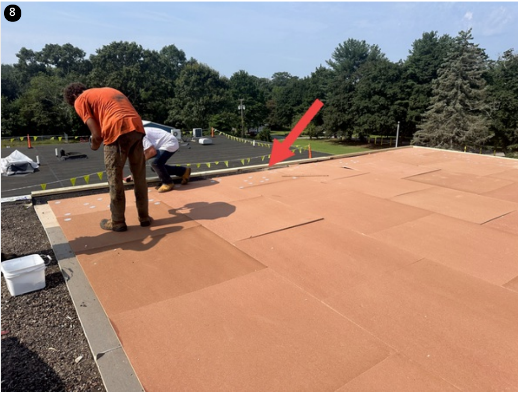
Overview of slope on upper roof section
