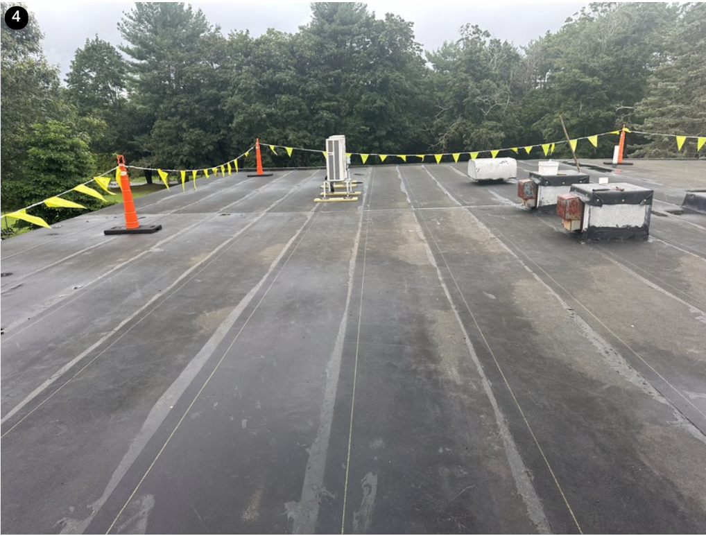
Last section on South wing ripped and base sheets installed
