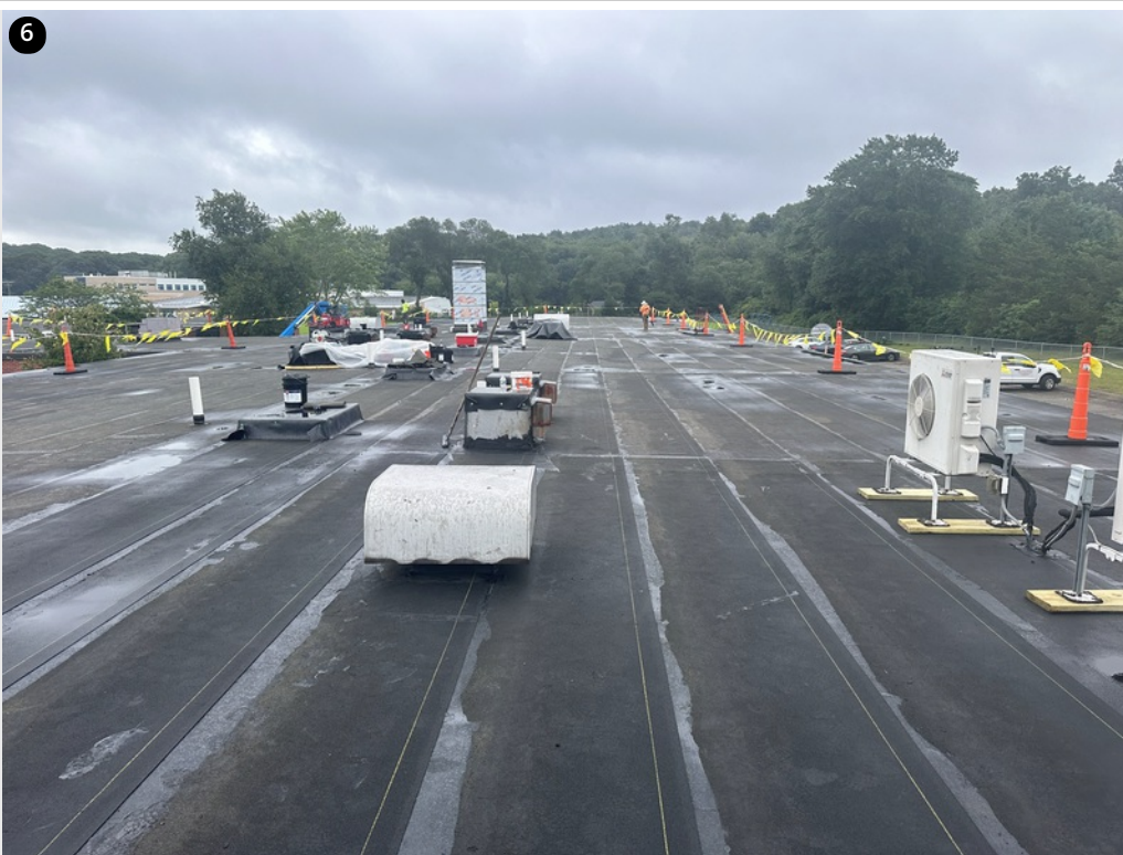
Overview- Completed base sheet installation on South wing
