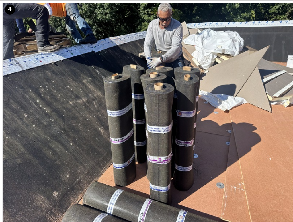
Base sheets being prepped for installation
