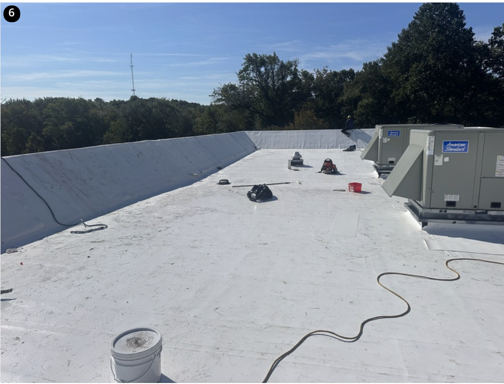
Overview- Cap sheet installed- Field seams heat welded- Curb flashings being prepared
