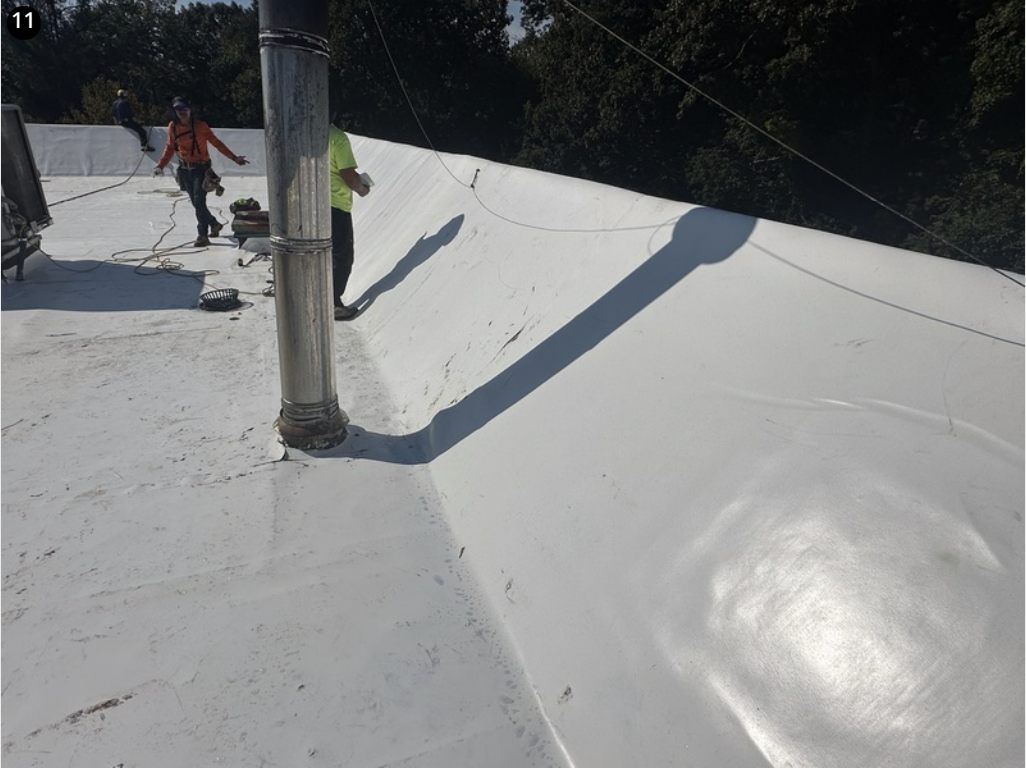
Cap sheets installed around stack
