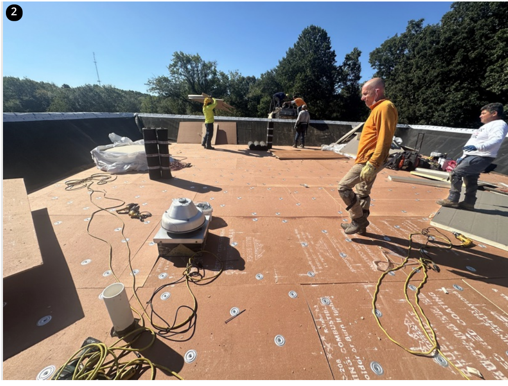
2 Crew laying out and fastening cover board to existing deck
