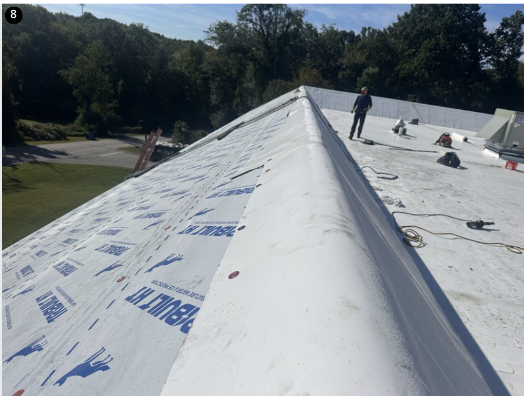
8 Cap sheets back nailed over ridge
