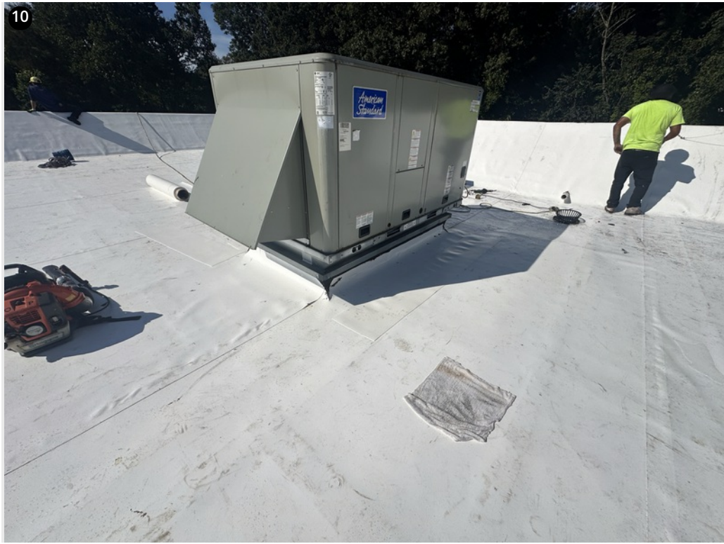
10 RTU- Curb flashings prepped
