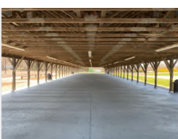
Concrete Floor Pole Barn Lower Town Green
