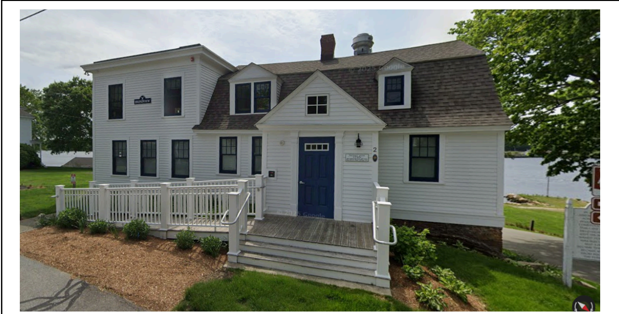
Cape - Thomas Geer House, c, 1796; large addition, c. 1890
