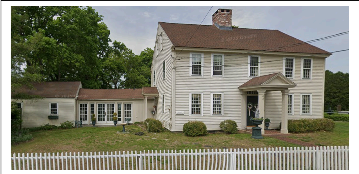
Federal - Daniel Copp House, c. 1796
