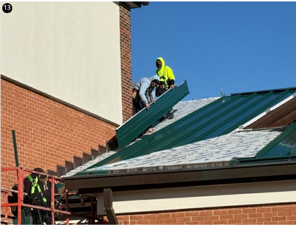
Crew installing panels near Gym- 12/13/24
