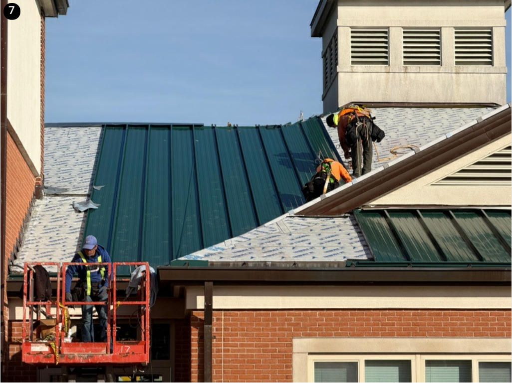
Crew installing panels behind copula- 12/9/24
