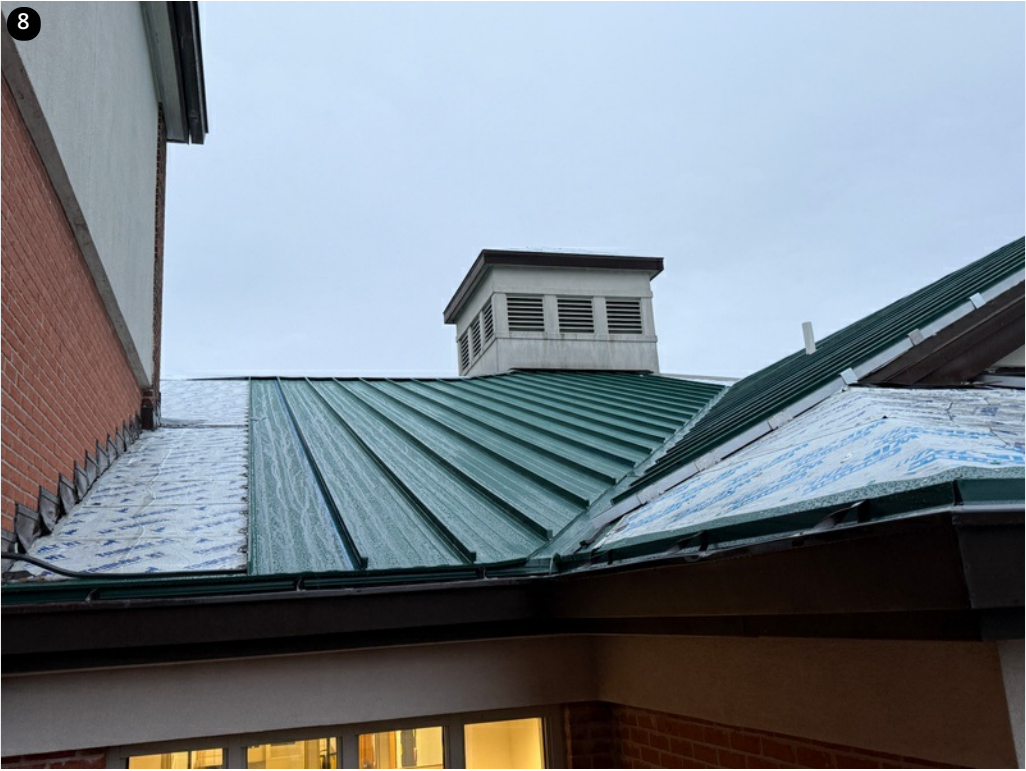
Overview- Panels installed behind copula- 12/9/24
