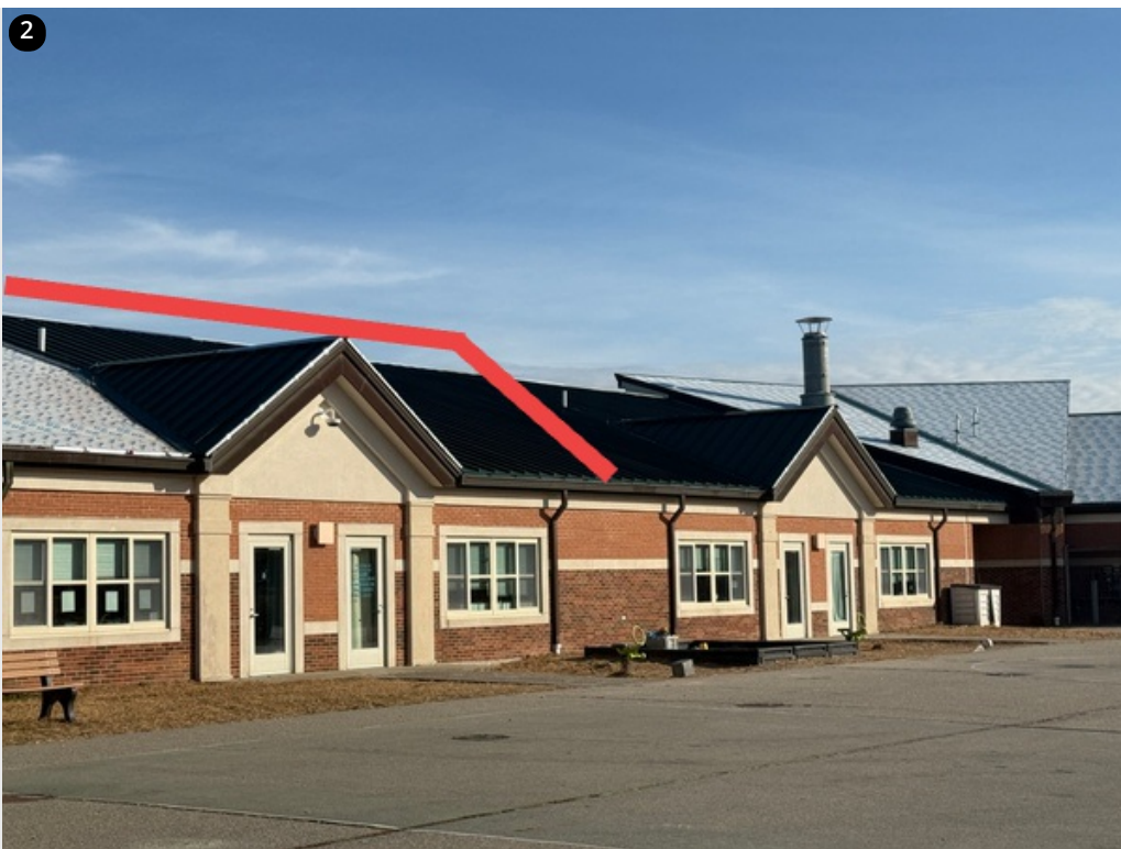
Panels installed up to second dormer on Saturday, 12/7/24
