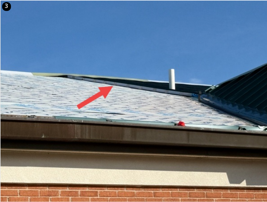
Overview of clip spacing on panels installed on 12/7/24
