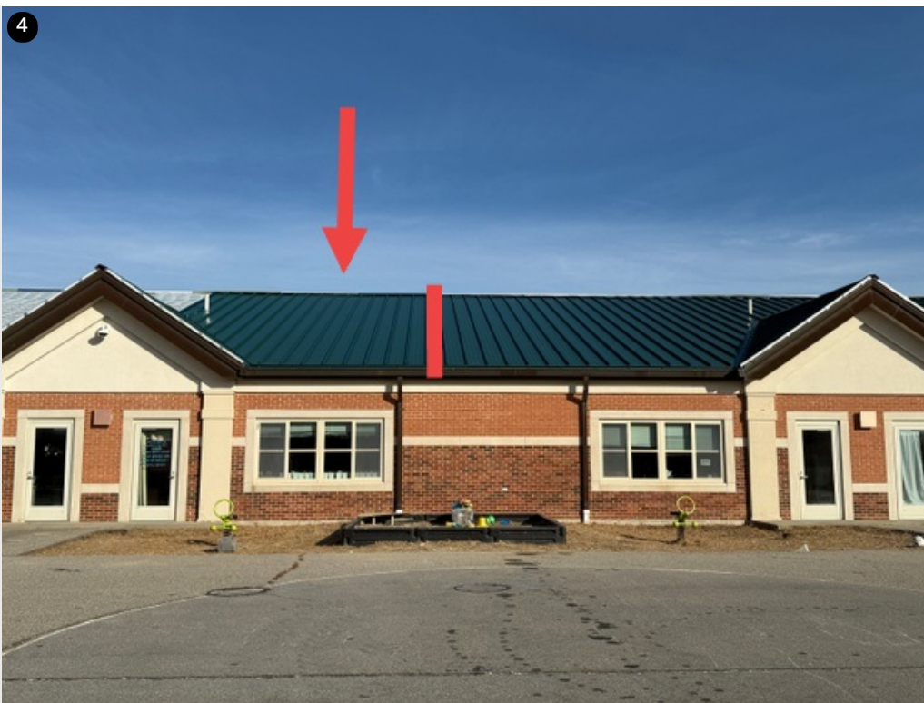
Overview- Panels installed Saturday, 12/7/24
