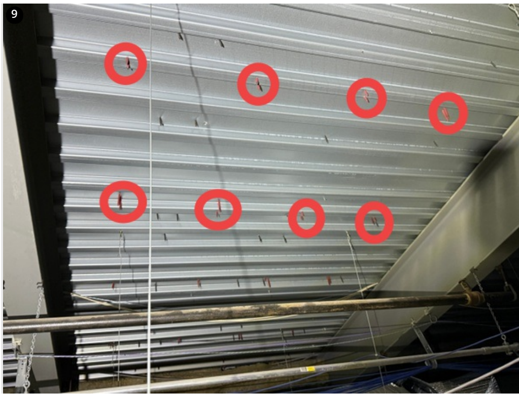
Fasteners observed penetrating roof deck- 12/9/24
