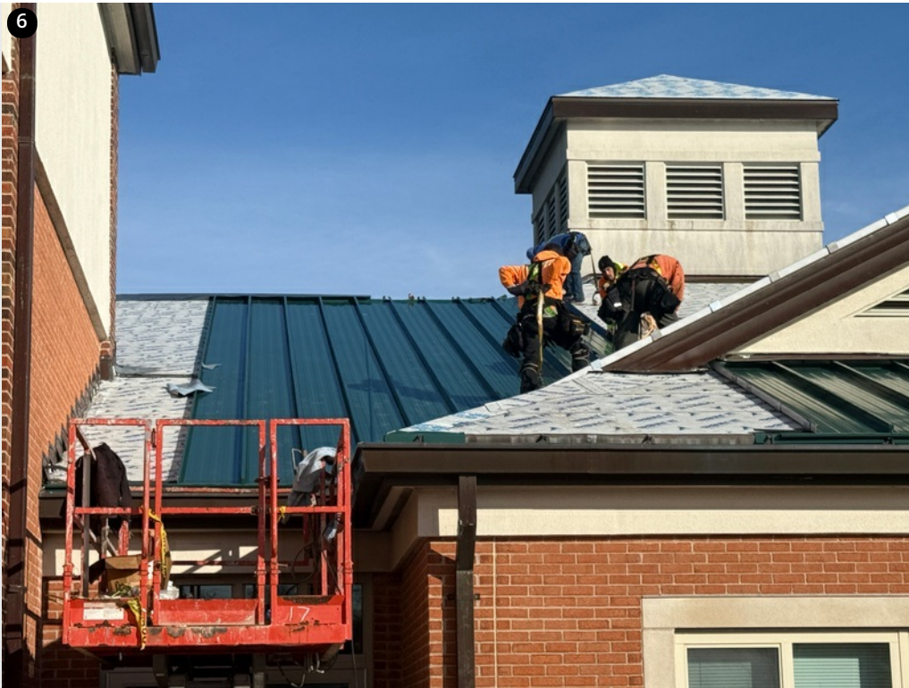
Crew installing panels behind copula- 12/9/24
