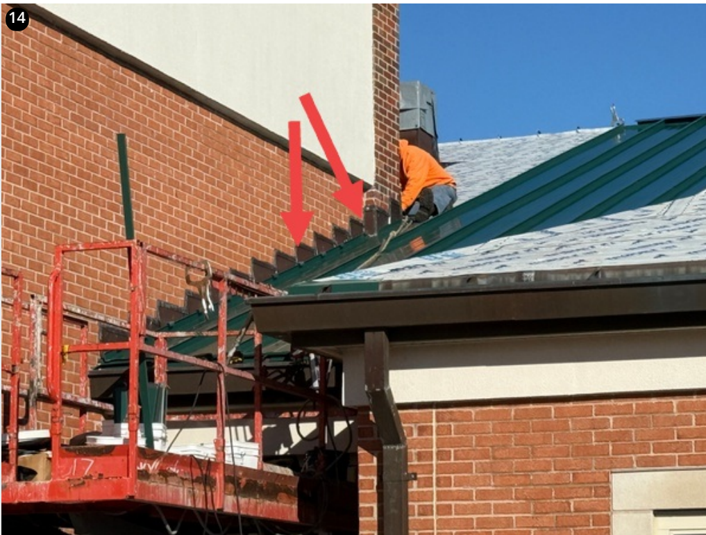
Panel field cut to match masonry bump out and installed- 12/13/24
