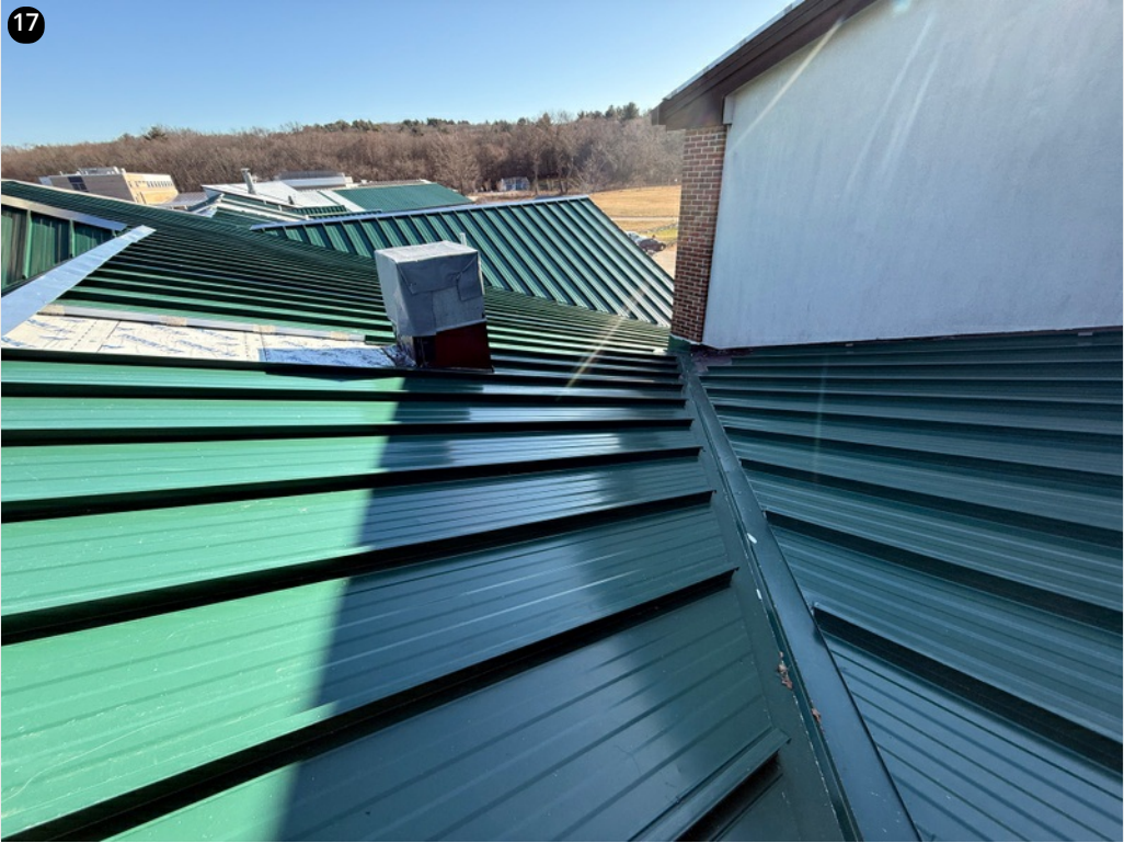
Panels installed in valley area- 12/14/24
