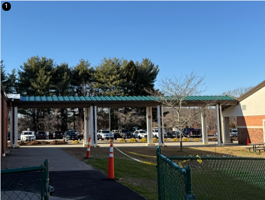
Walkway roof completed- 12/7/24
