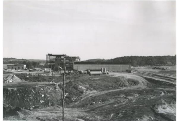
Site under development as Dow Chemical Plant
