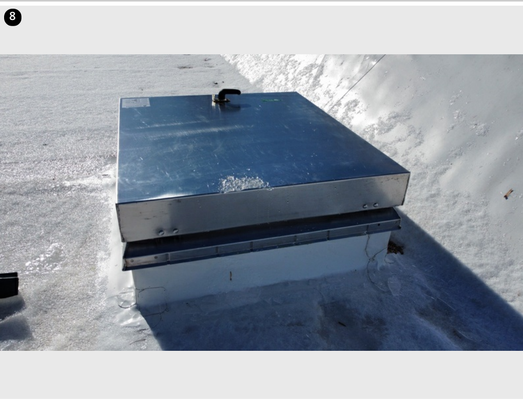
New roof hatch installed- 12/4/24
