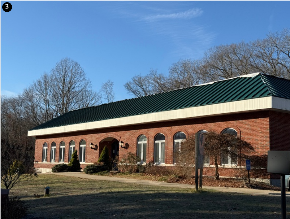
Completed East side roof section- 12/2/24
