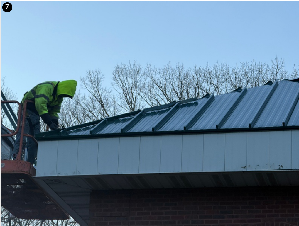
Crew installing head closures on South East corner
