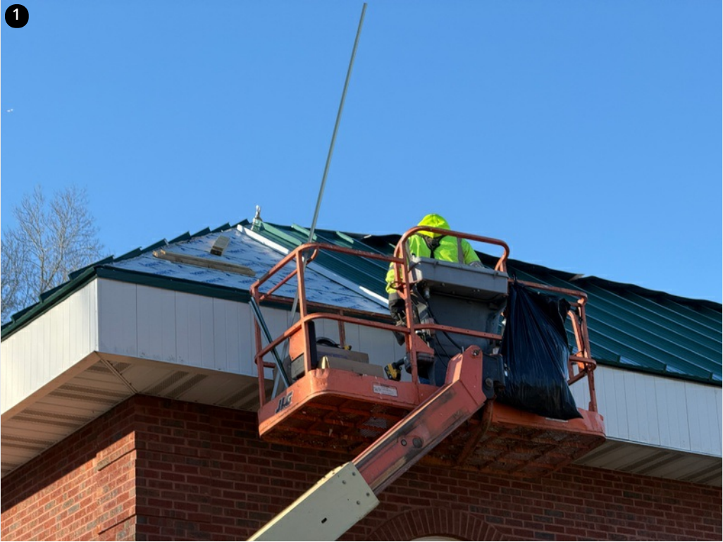
Crew finishing install of panels on East side roof section- 12/2/24
