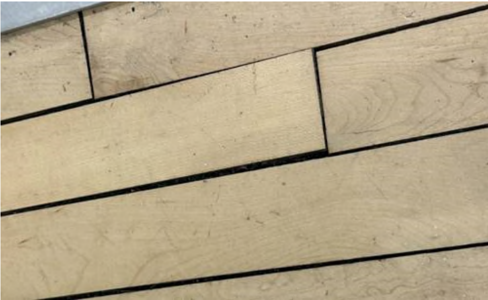
Floor boards separating and even breaking apart.
