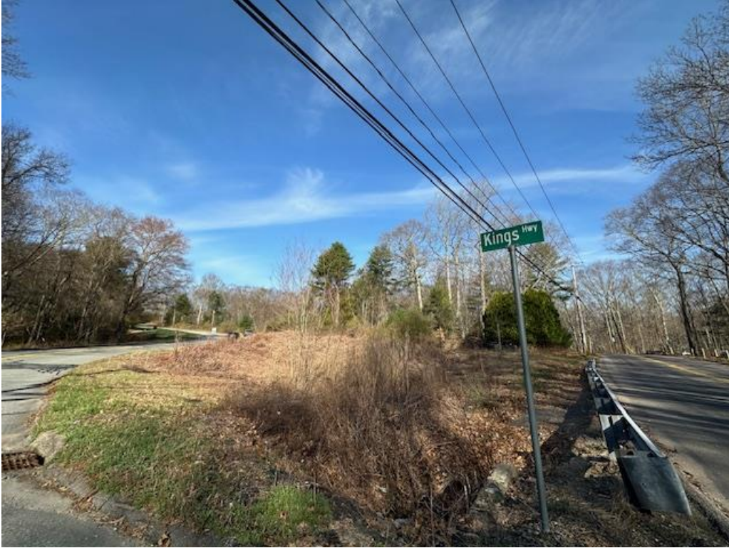
Photo 1: Example of the wetland conditions of the detention basin at the corner of Kings Highway and Christy Hill Road.
